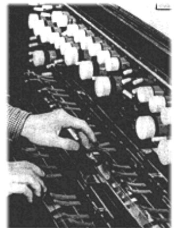
**fig. 39** The Mixturtrautonium showing the resistance wires with leather thongs.
