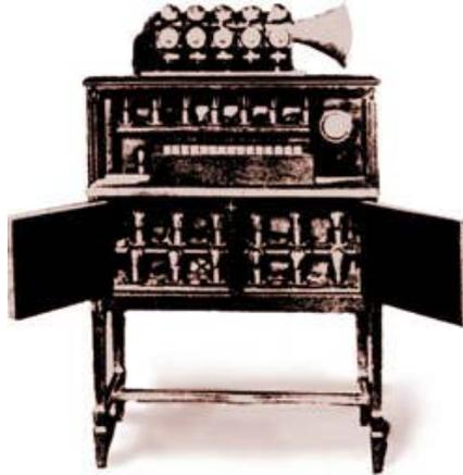
fig. 26 The Pianorad, showing oscillators and speaker horn
