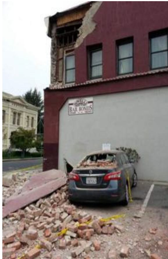
Figure 2-4. Damage to an unretrofitted URM building in the 2014 South Napa earthquake. Adjacent buildings were temporarily closed until this building could be secured. Photo: J. Maffei
