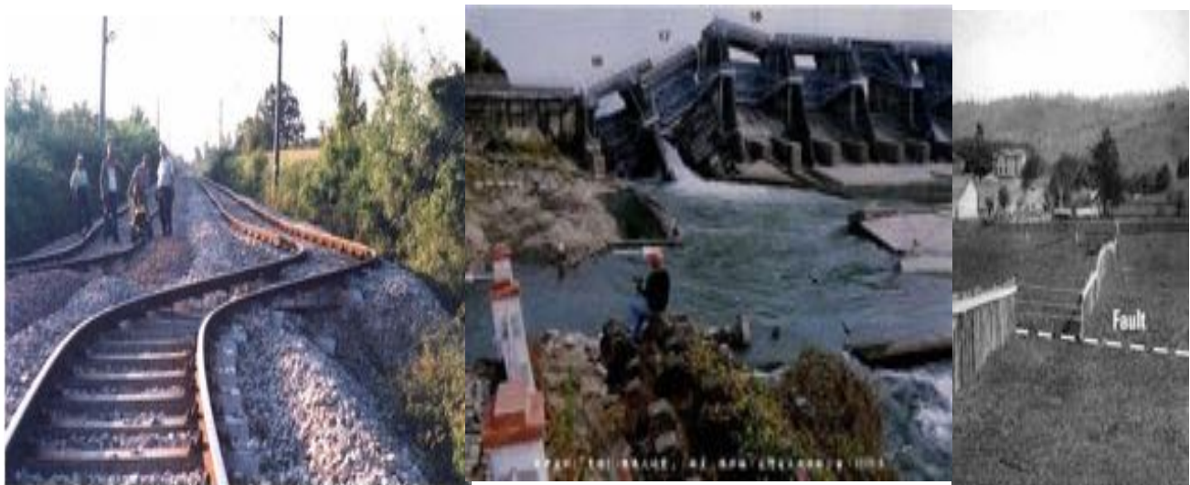
Figure 3-4. Three examples of fault crossing damage. The railway was bent when the fault in the 1999 Izmet, Turkey earthquake moved sideways (lower part of the picture to the left) about 7 ft. The dam was damaged when the 1999 Chi Taiwan earthquake moved (right side up) about 25 ft. The fence was broken when the 1906 San Francisco earthquake moved 5 ft.
