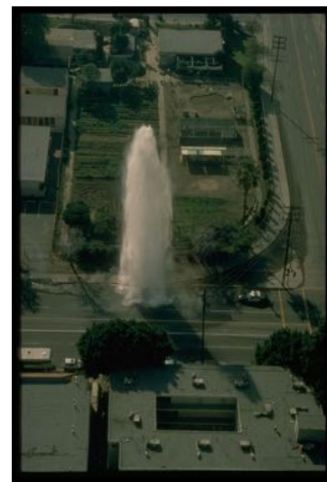
Figure 3-5. Geyser from a broken water main in the 1994 Northridge earthquake.
