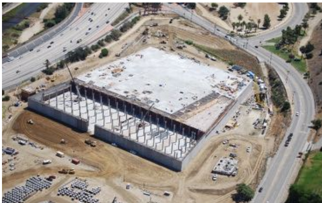
Fig. 3-6. An aerial photograph of the Headworks Reservoir during construction.
