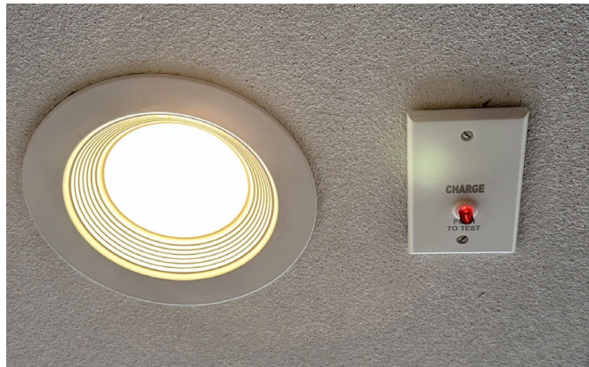
Figure 2: Test button and LED indicator provided for the adjacent general-purpose downlight fixture with battery backup. Courtesy: SHP
