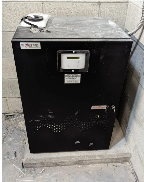
Figure 3: An installed emergency lighting inverter. Courtesy: SHP
