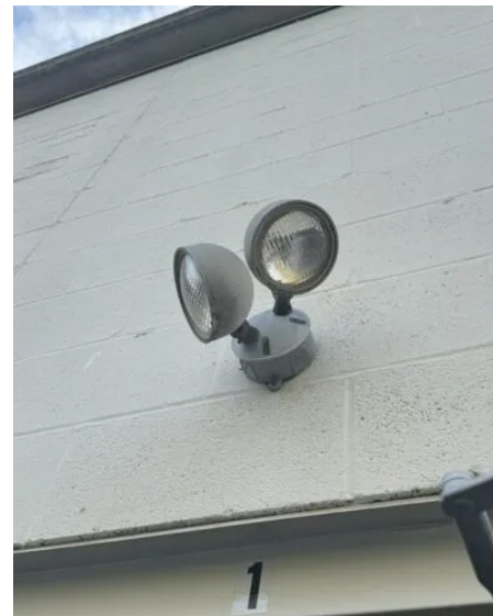
Figure 4: Exterior rated unit battery supplied lighting. Batteries are located on the interior of the building. Courtesy: SHP
