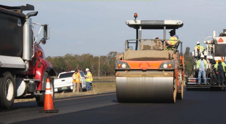
he Alabama Department of Transportation(ALDOT) is conducting an experiment on a four-lane highway involving an advanced, non-toxic asphalt rejuvenator in a pavement mix
