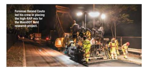
pavement may experience an early onset of premature cracking due to the stiffness of the aged binder. Industry can offset that brittleness by using a softer binder grade or rejuvenators. Mogawer was using the Delta S rejuvenator in the lab; now it needed to be put to test in the field. MassDOT District 3 and P.J. Keating opted to use it for a pavement in Worcester."
