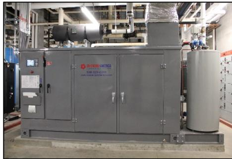
**Figure 7-7. Energy Choice EC 190 Natural Gas system, 190 kW**
