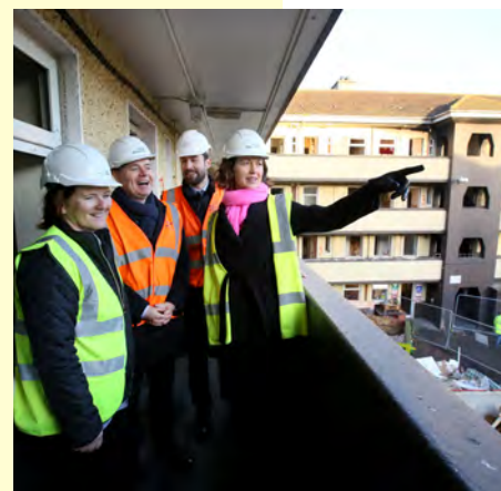
Refurbishment of Mary's Mansions
