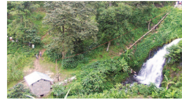
The Intermediate Technology Development Group (ITDG) has installed very small 'pico hydro' for communities living on Mount Kenya. The power plants generate electricity for lighting, radios and mobile phone charging. Pico hydro does not generate enough energy for cooking, however.
