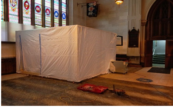
Dust containment tent with filter/fan attached
