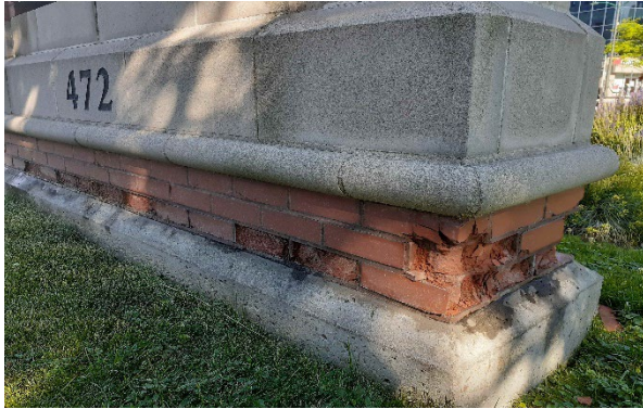
Deteriorated masonry
