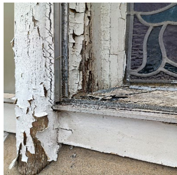
Wood rot and paint deterioration
