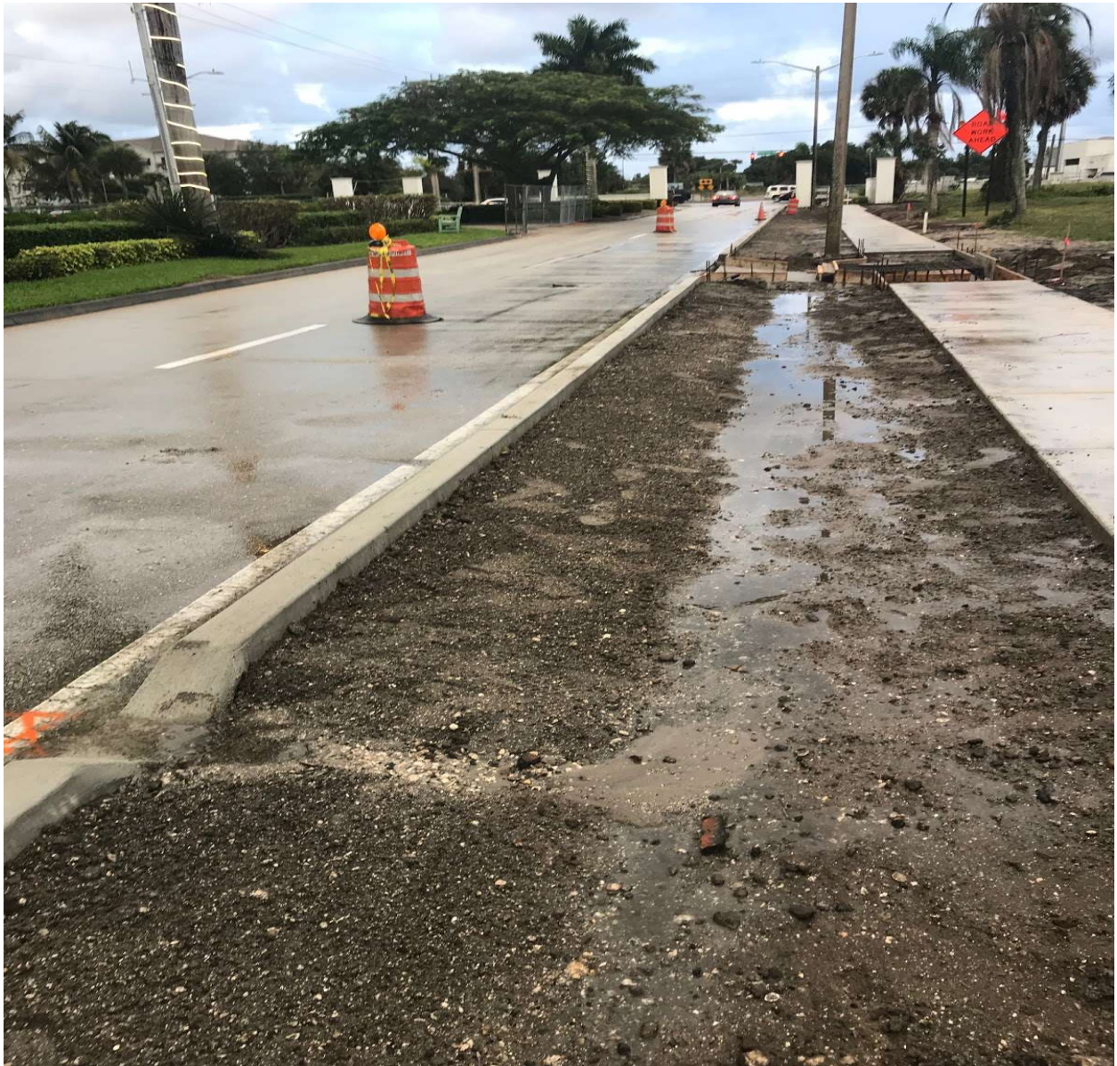
CENTURY BOULEVARD- CURB INSTALLATION COMPLETE, RAIN WATER FROM ROADWAY MOVING TO DRAINAGE SWALE BETWEEN SIDEWALK AND CURB.
