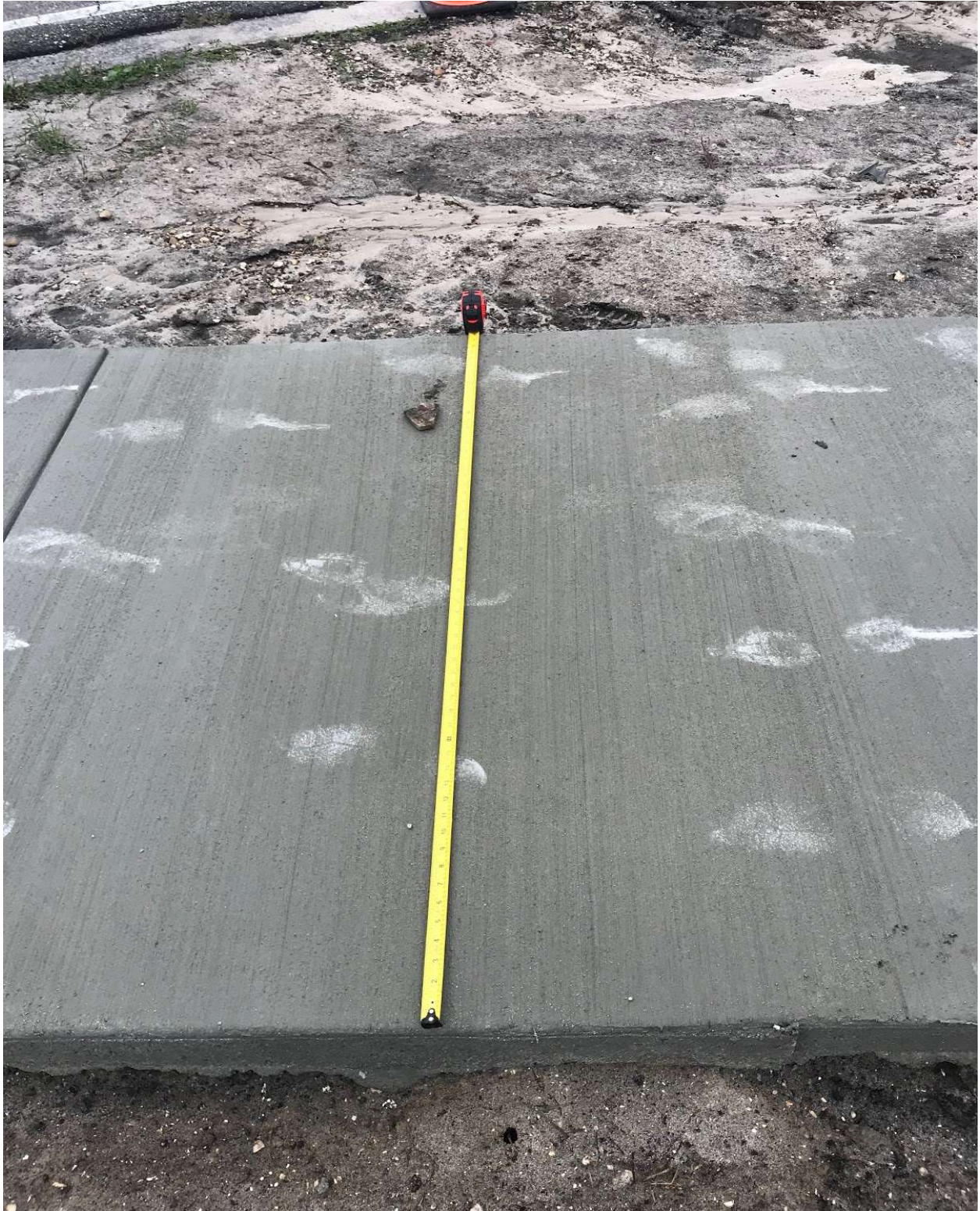
CENTURY BOULEVARD- WALKWAY IS MINIMUM FIVE FEET WIDE, AS PER ENGINEER'S SPECIFICATIONS.
