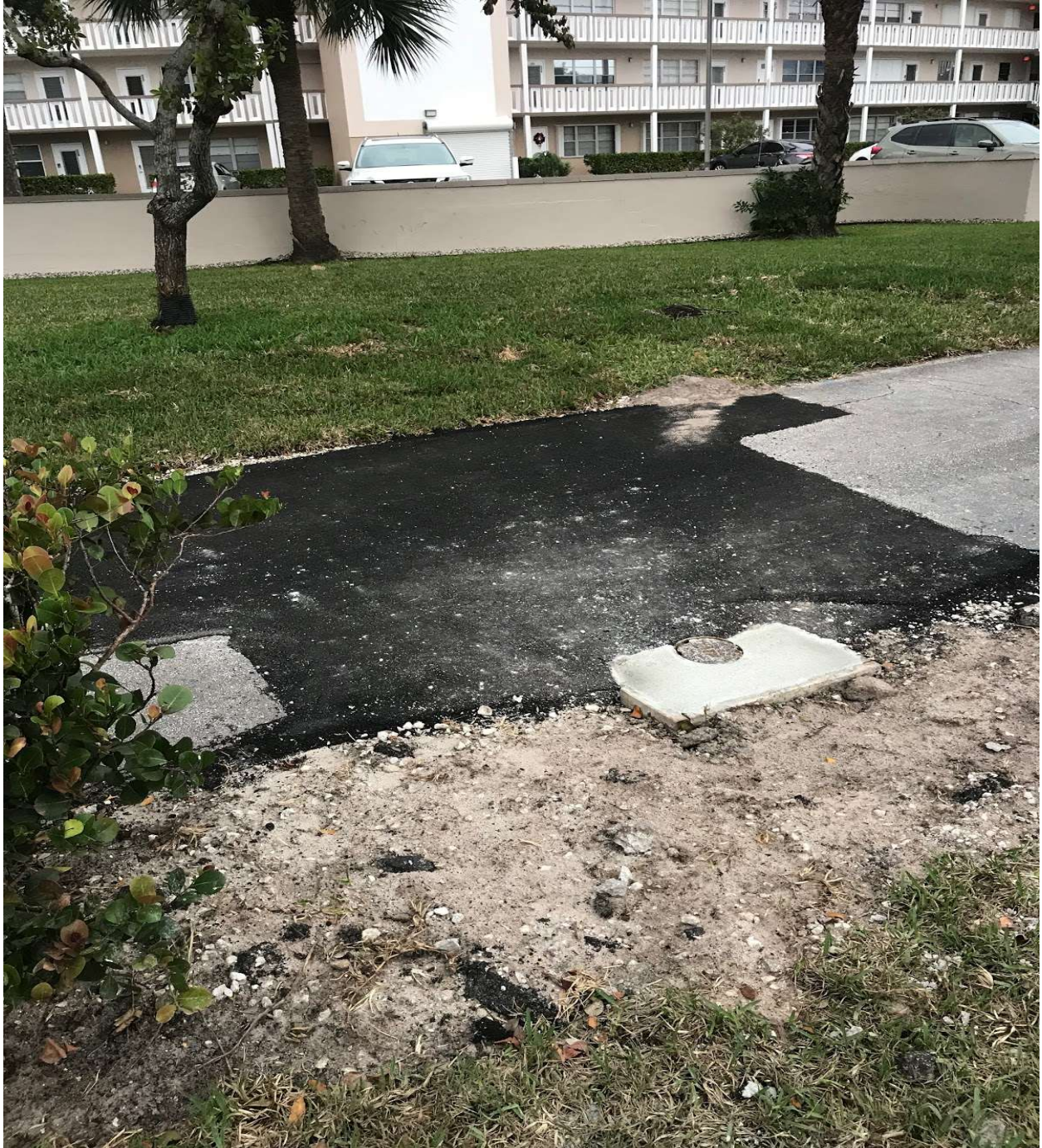
DOVER SECTION- INCOMPLETE PAVEMENT REPAIR AT SOUTH DRIVE WALKWAY. ADDED TO PUNCH LIST.
