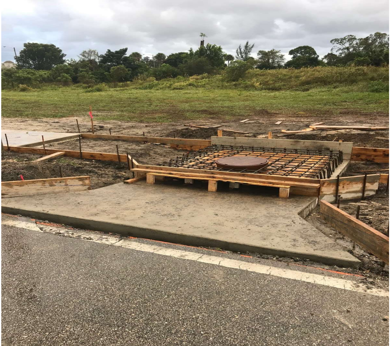
CENTURY BOULEVARD- EASTERN DRAINAGE FLUME READY FOR CONCRETE POUR.
