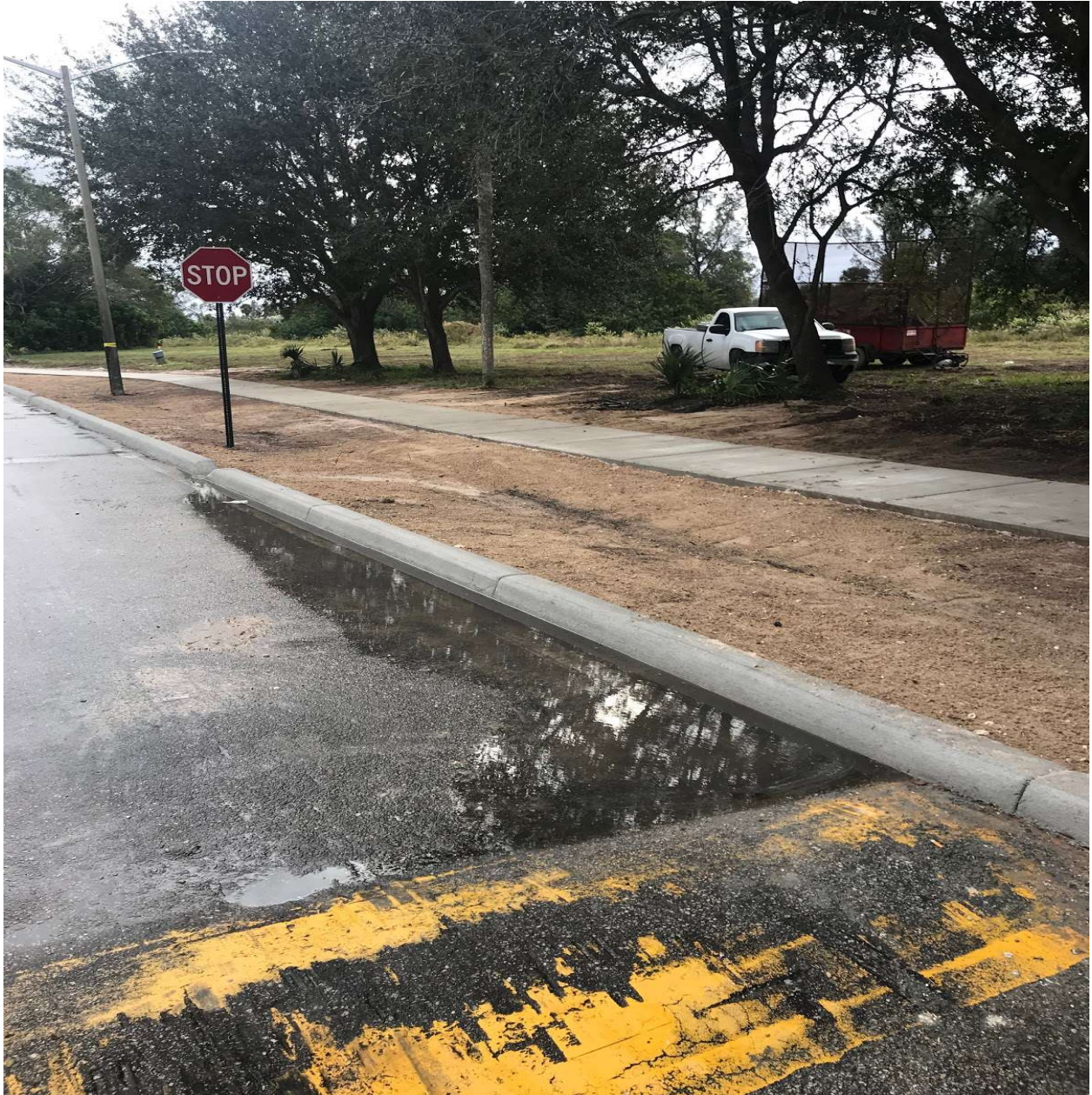
CENTURY BOULEVARD- WATER COLLECTING AT JUNCTURE OF NEW CURB AND SPEED BUMP. THIS WILL BE ADDRESSED BY AN ADDITIONAL CURB CUT. ROADWAY STRIPING AND SPEED BUMPS WILL BE PAINTED AFTER PROJECT IS COMPLETE.
