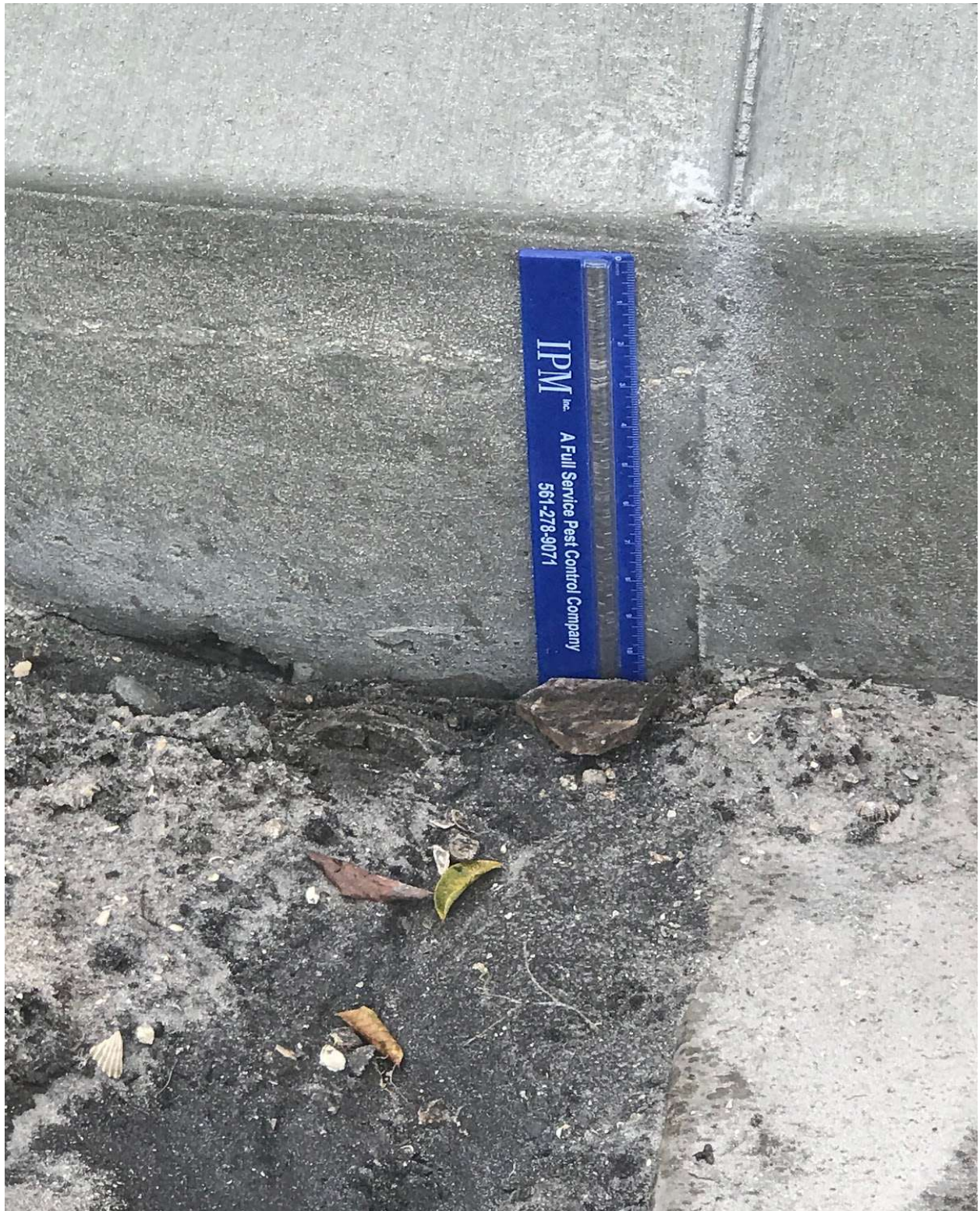
CENTURY BOULEVARD- SIDEWALK AT DRAINAGE FLUMES IS TWELVE INCHES THICK, AS PER ENGINEER'S SPECIFICATIONS.
