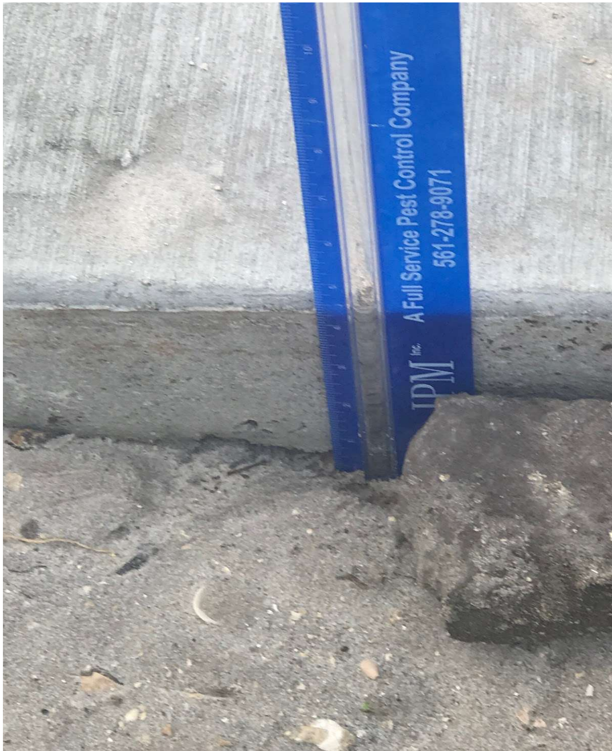
CENTURY BOULEVARD- SIDEWALK IS MINIMUM FOUR INCHES THICK, AS PER ENGINEER'S SPECIFICATIONS.
