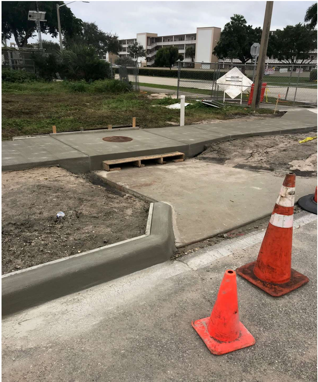
CENTURY BOULEVARD- CONCRETE POUR AT WESTERN DRAINAGE FLUME COMPLETE.
