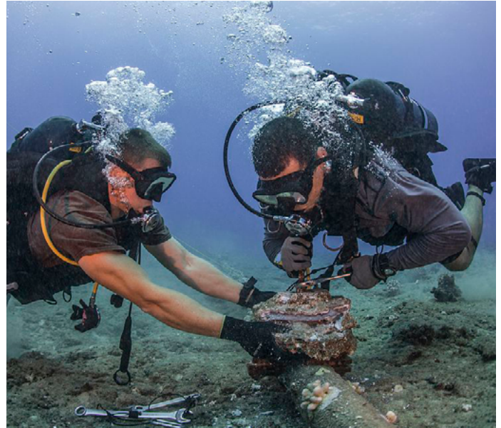
Members of an underwater construction team repair an undersea cable. Photo: Charles E. White, U.S. Navy.
