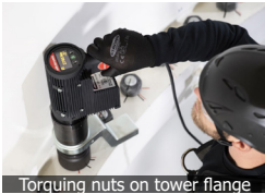
Torquing nuts on tower flange
