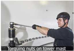
Torquing nuts on tower mast
