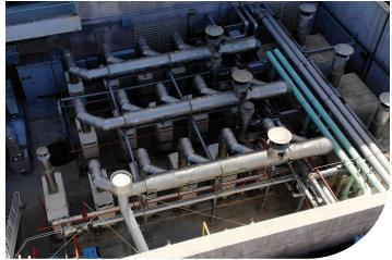
Natural gas-fired microturbines generate nearly all of the building's electricity, while capturing the process heat to operate absorption chillers for energy-efficient cooling or space heating.
