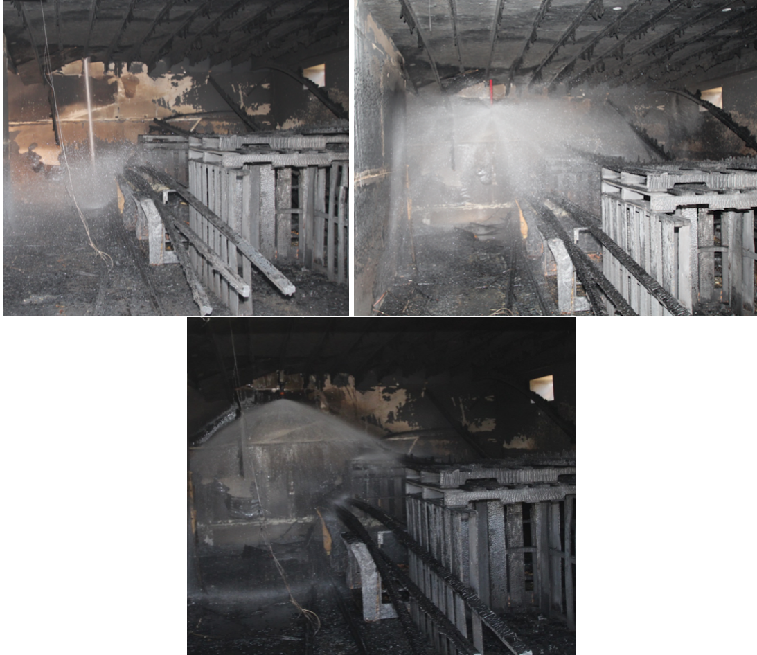
Figure 6.14: Photograph of straight stream (top left), the 150 gpm piercing nozzle (top right), and fog stream (bottom) flowing through a hole punched through the floor.
