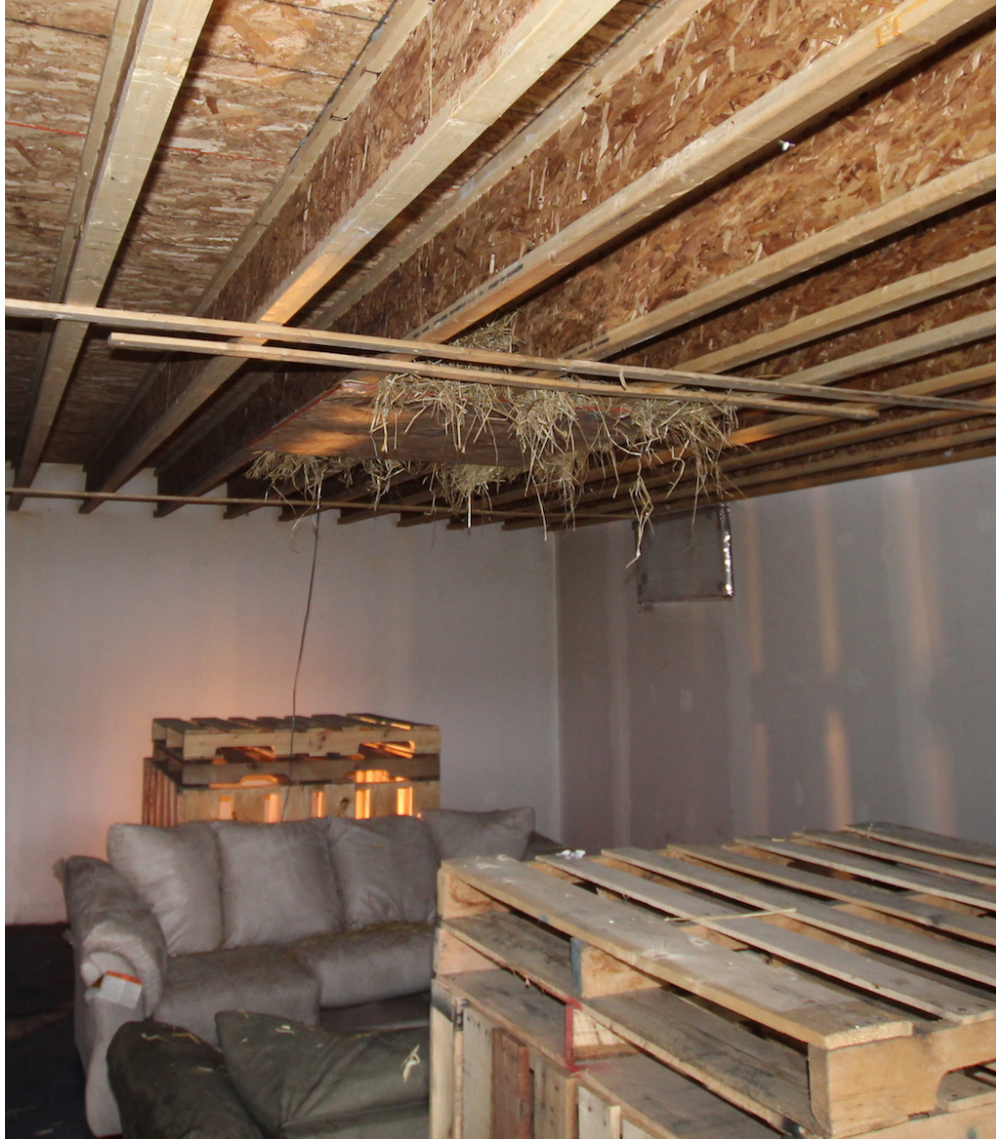
Figure 3.7: Photograph of hay and OSB installed between I-joists for an experiment with a ceiling ignition.
