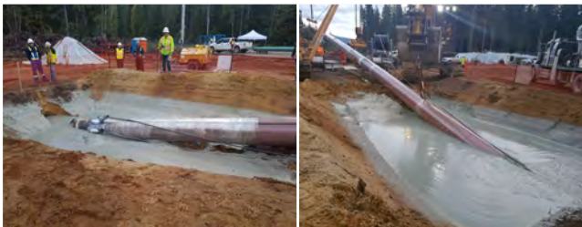
Figure 3. Trenchless Crossings – Horizontal Directional Drills (HDD).
