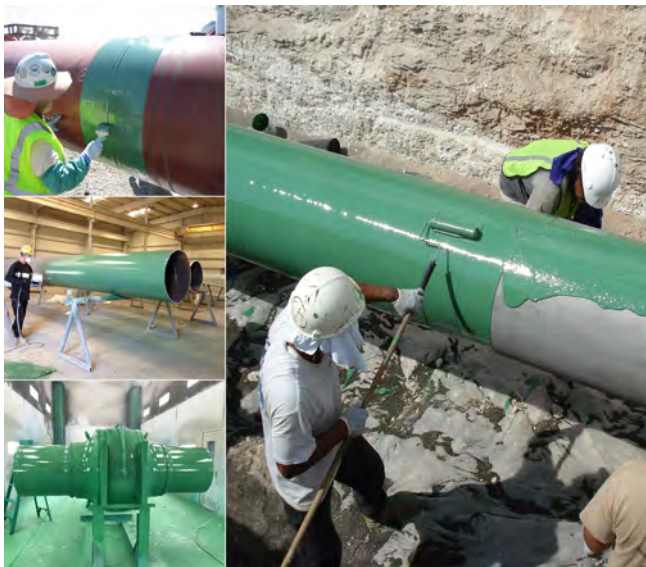
Winn & Coales International Ltd. Protal 7200™ can be easily applied by brush, roller or spray in high and low temperature environments.
