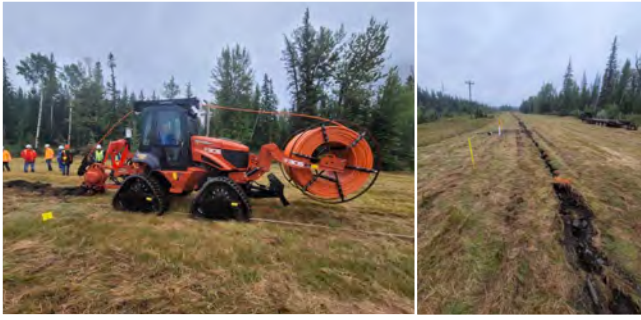
Figure 5. Trench-based retrofitting of existing pipeline segment.
