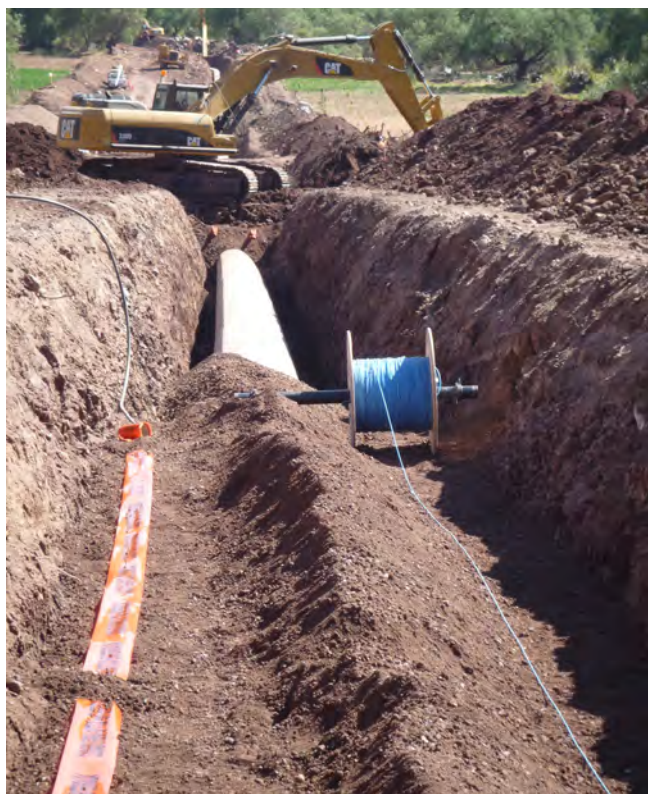
Figure 1. Fibre optic cable laying for CO 2 pipelines.
