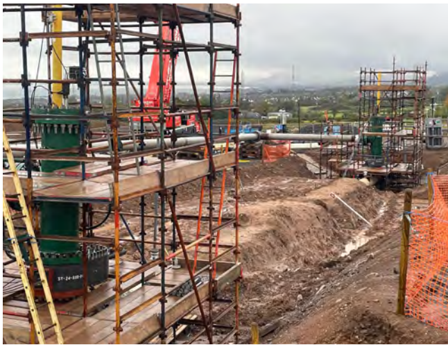
Figure 2. 24 in. Dual BISEP and integrated bypass, gas pipeline tie-in (Northern Ireland, UK).
