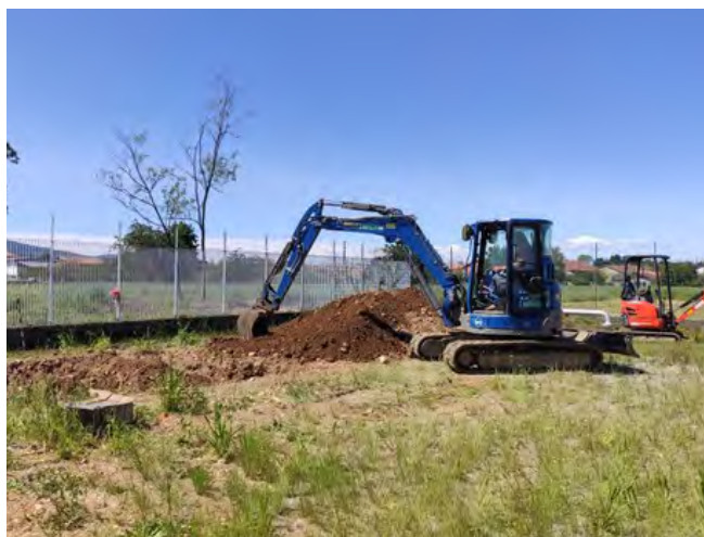
Figure 5. Mechanical excavation performed to calibrate the e-vpms TPI detector.
