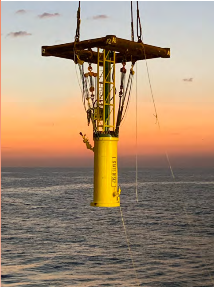
Figure 1. 48 in. Subsea BISEP deployment, (Arabian Gulf).
