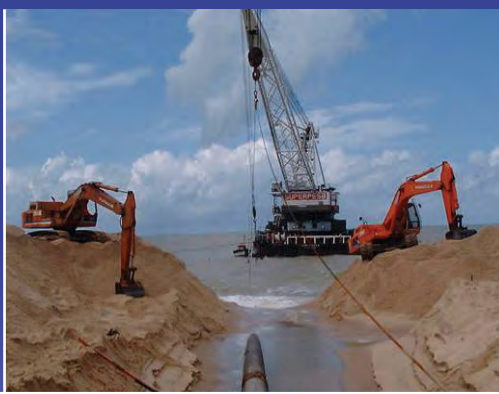
Brasil Post Trenching Rough Shore Approach (Lead Keel Machine)
