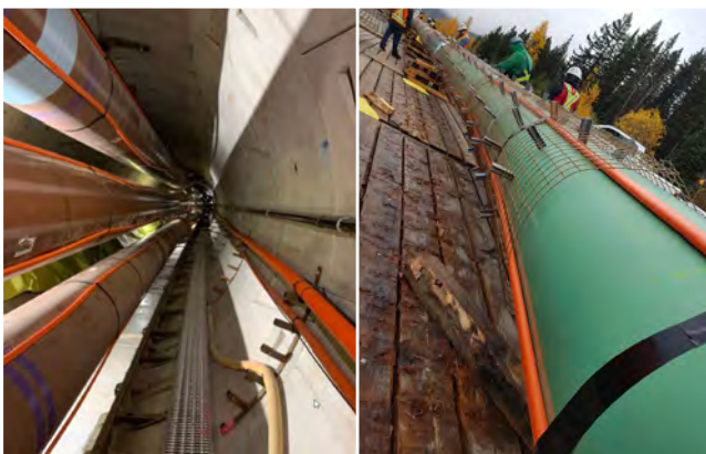
Figure 4. Burnaby tunnel deployment and concrete casing preparation.
