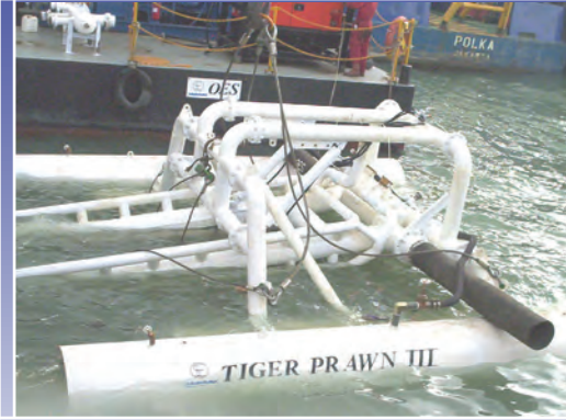
Floating Jet Sled across mud flats too shallow for barge
