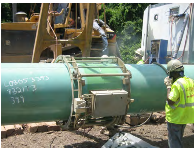
Winn & Coales International Ltd. Application of Protal 7200 in the field.
