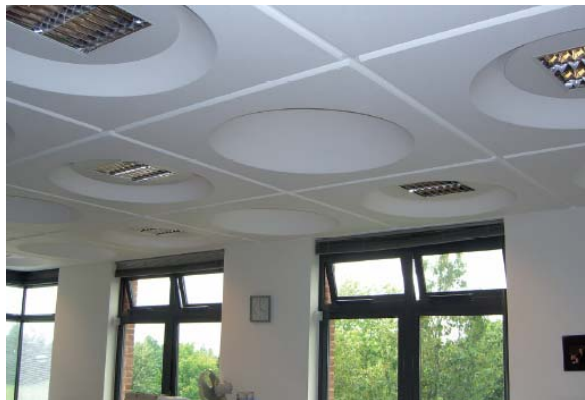
Figure 11.6 – inside the building
