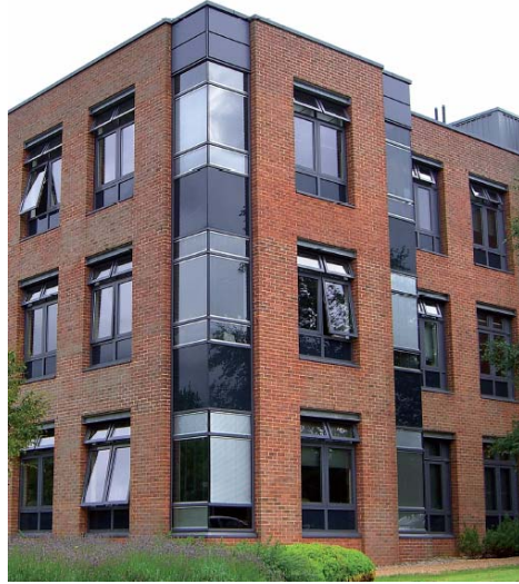
Figure 11.5 – Charities Aid Foundation building
