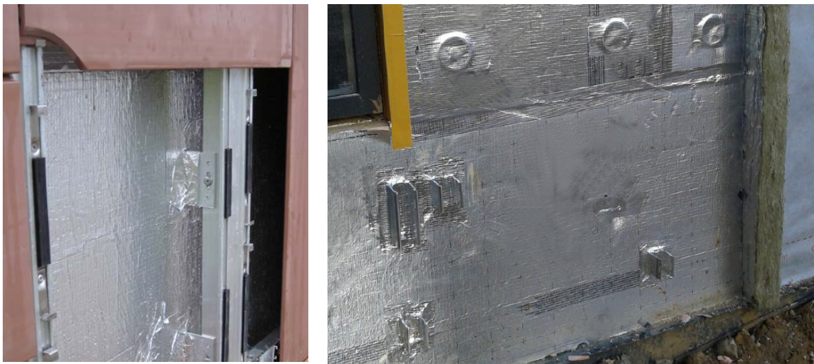
Figure 5.12 – Foil faced insulation as water barrier
