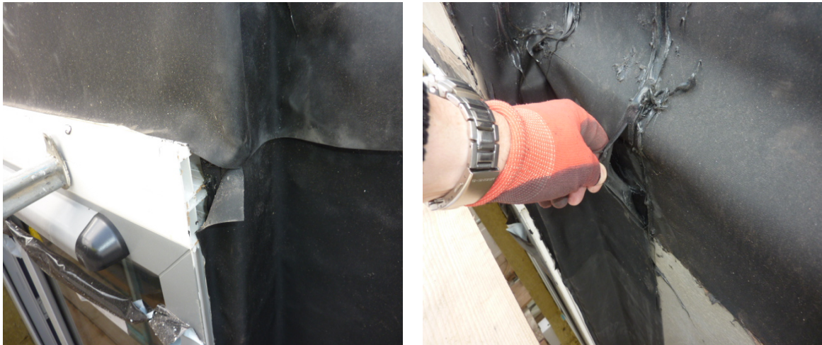
Figure 5.5 - Membrane seals around windows
