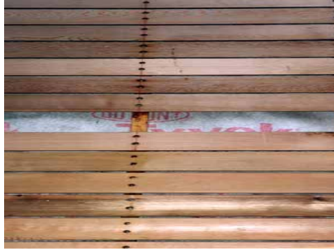
Figure 4.14 - Breather membrane behind a timber rainscreen
