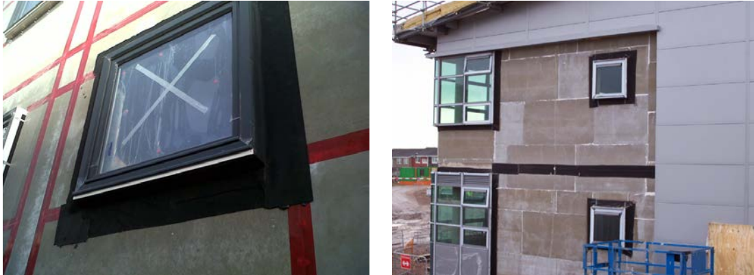
Figure 5.4 - EPDM membrane between window frame and sheathing
