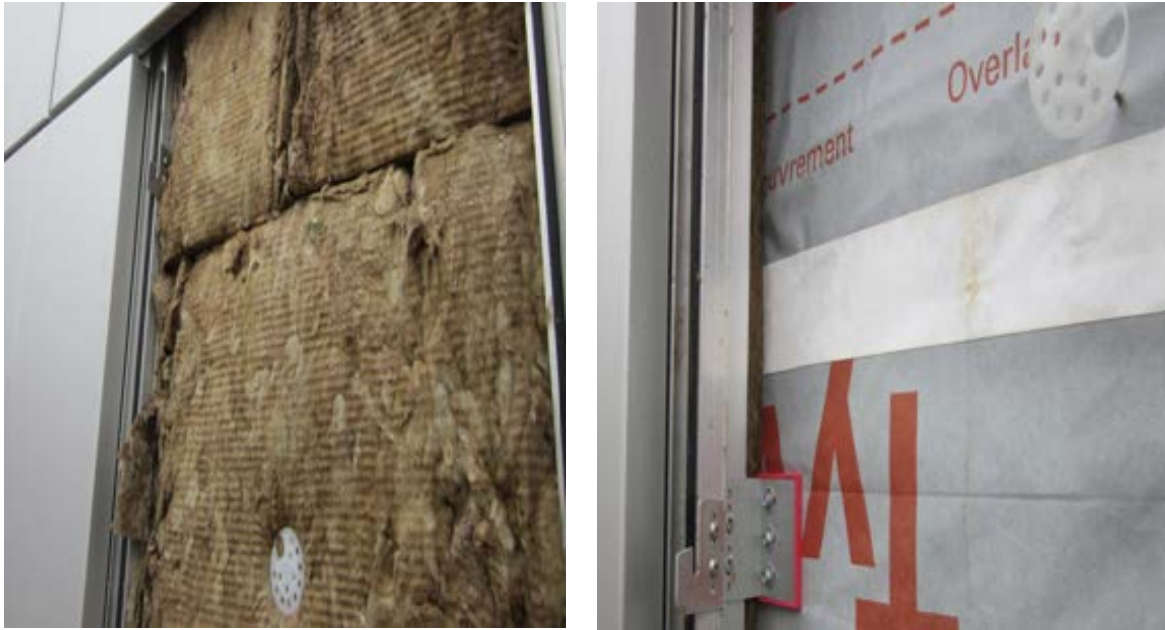
Figure 4.20 – Typical insulation fixings in a rainscreen system
