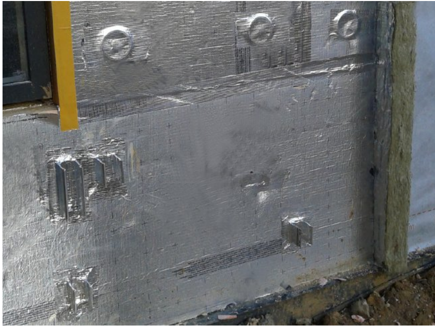
Figure 4.19 – Foil face insulation boards, taped joints and bracket penetrations
