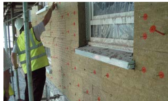
Figure 1.3 - Different components of a built-up wall (rainscreen (left), external insulation (right))
