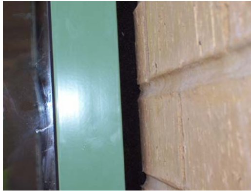
Figure 5.7 - Sealant and backer rod (left), foam sealing tape (right, ©STO), impregnated foam tape seal between window and brickwork wall (bottom)
