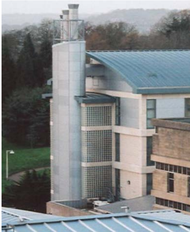
Figure 7.7- Repaired metal panels
