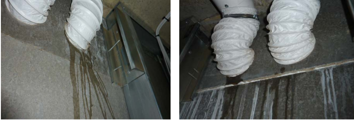
Figure 5.31 - Service penetration through the backing wall
