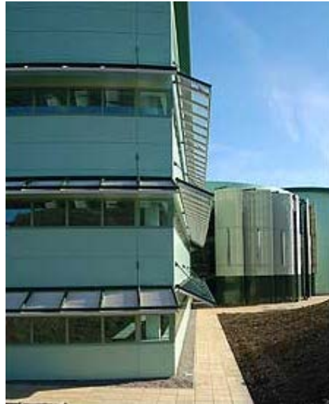
Figure 5.33 - Shading devices fixed to a rainscreen wall
