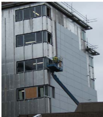
Figure 1.3 - Different components of a built-up wall (rainscreen (left), external insulation (right))
