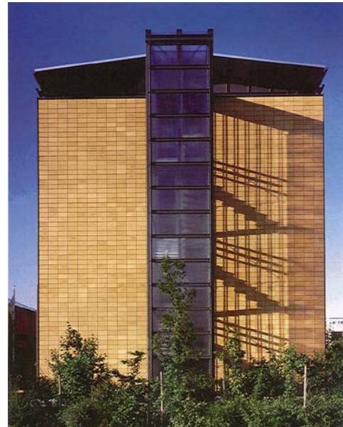
Figure 1.10 - Built-up walls – insulated render and rainscreen systems
