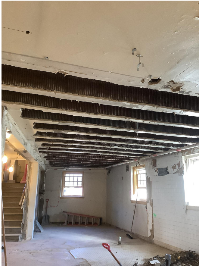
Plaster Ceiling Removed & Concrete Slab Exposed
