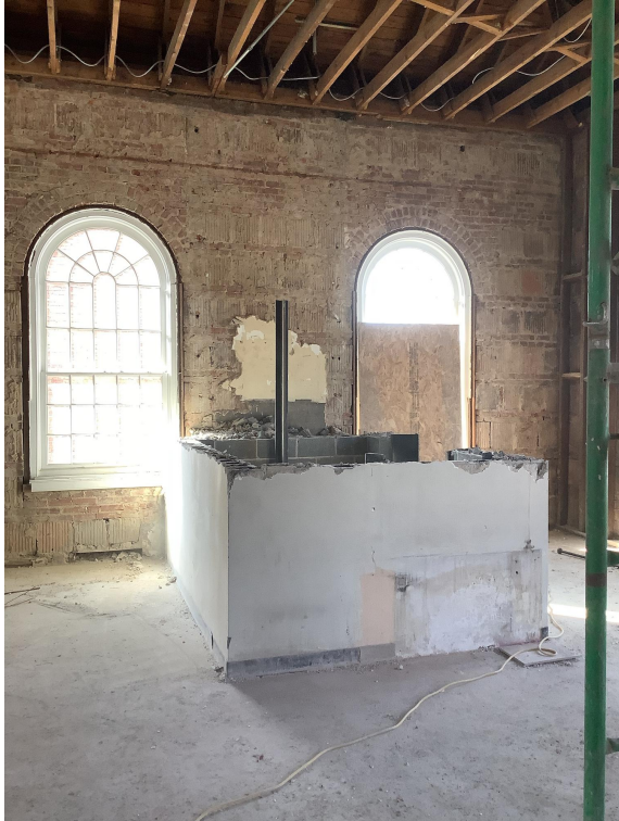
Demolition of Existing Elevator & Shaft
