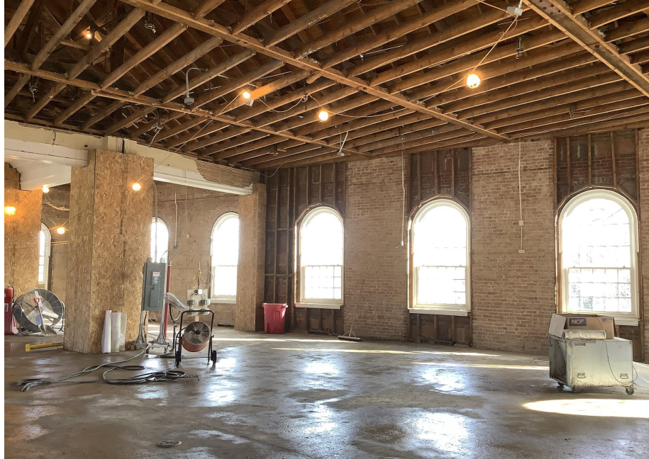
Ceiling Stripped Interior Walls Exposing Terracotta and Brick
