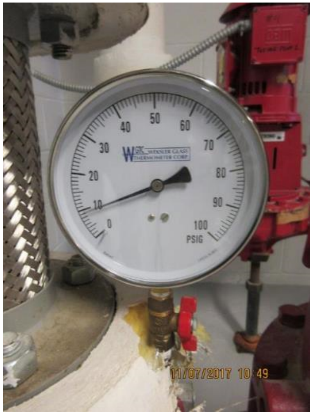
Lower Pressure Before the Pump Higher Pressure After the Pump
