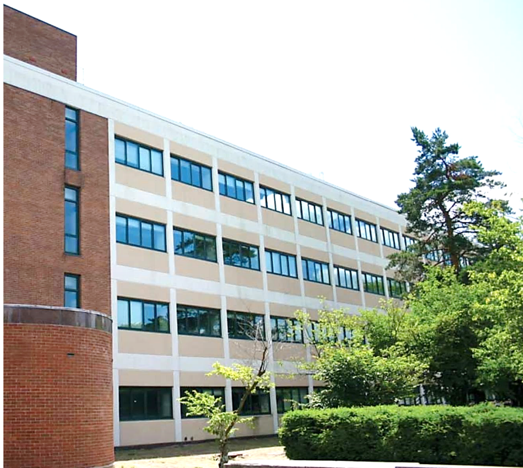
Coykendall Science Building
