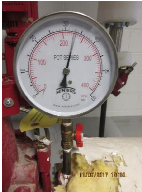
Lower Pressure Before the Pump Higher Pressure After the Pump
