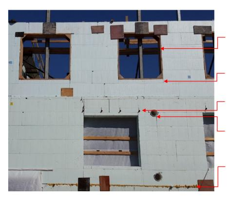
Integral cast insulated jamb are cleanest tightest detail
