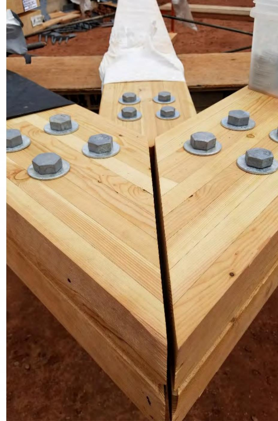
Embedded steel elements unite mass timber elements through bolted connections.
