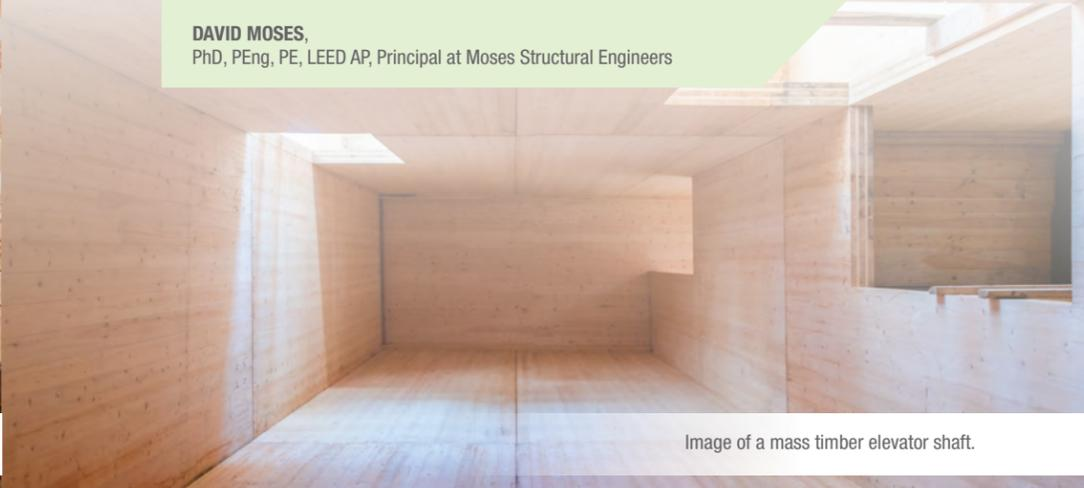
Image of a mass timber elevator shaft.
