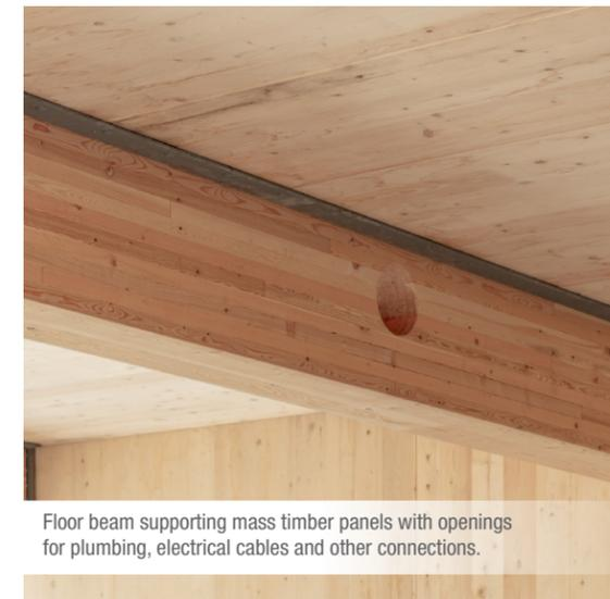
Floor beam supporting mass timber panels with openings for plumbing, electrical cables and other connections.
