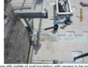
Areas still visible of roof insulation with pavers to be installed
