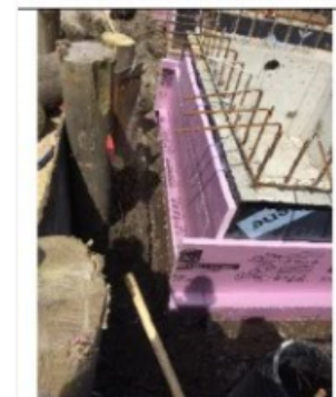
Insulation at grease trap area prior to backfill
