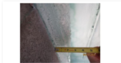
Thickness measurement, 2' spray foam at vertical
