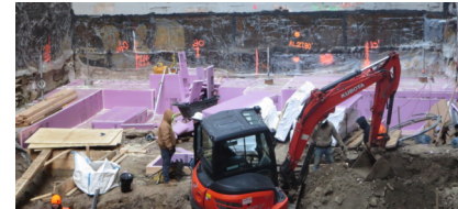
Below Grade Inspections
