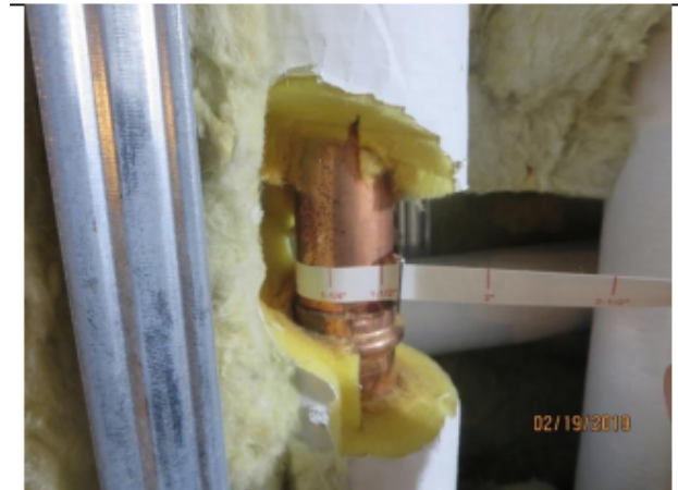
1.5" diameter hot water piping observed with only 1.0" thick insulation, 9 th floor
