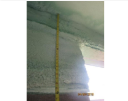
Thickness measurement, insulation extending down vertical 3'
