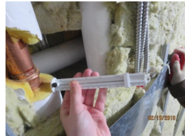
1.5" diameter hot water piping observed with only 1.0" thick insulation, 9 th floor
