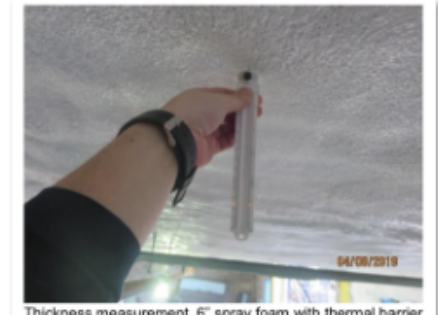
Thickness measurement, 6" spray foam with thermal barrier coating at horizontal
