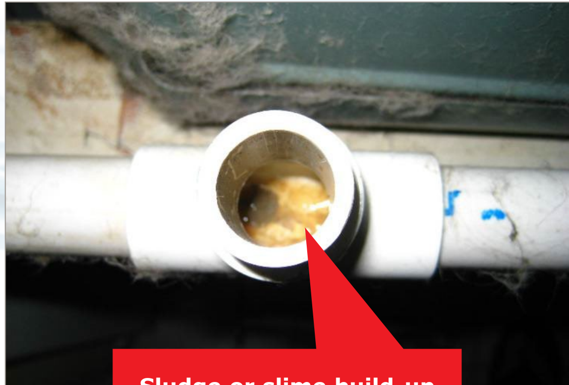
Sludge or slime build-up
