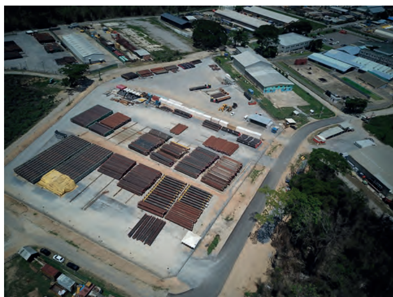
Figure 2. Granwood pipeyard in Chaguaramas, Trinidad.
