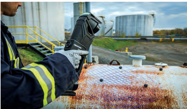
Figure 5. Accurate results and in-depth analyses directly onsite helps to establish valid diagnoses and orient repair decisions.
