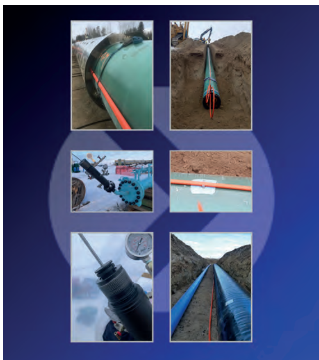
Figure 2. Deployment types of fibre optic cable.
