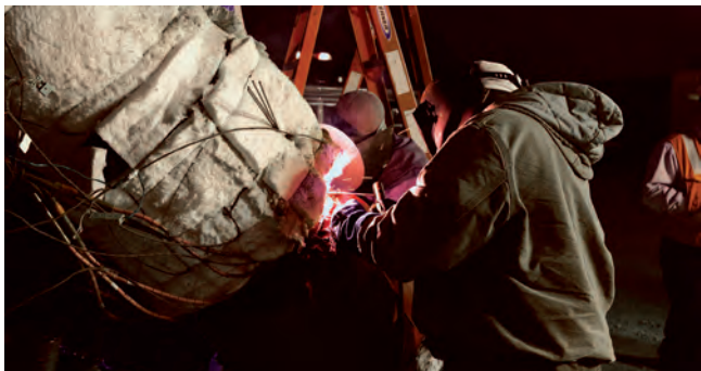
Figure 4. Heating blankets used to preheat the fitting and pipeline to proper temperatures during simulation at the test loop.
