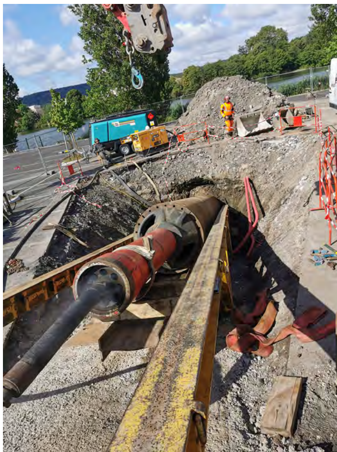
Figure 2. A double T-beam ensures safe guidance of the rammer in the soft bank soil. The add-on cone connects the Goliath firmly to the steel pipe.
