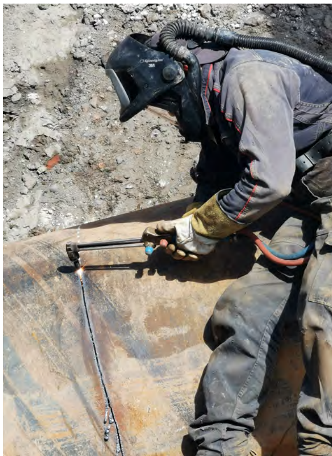
Figure 1. The 6 m long steel pipes for the 30 m long casing were welded on individually during the installation process.
