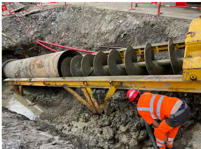
Figure 3. Once the ramming is done, the accumulated soil is removed from the casing pipe using an auger drill.
