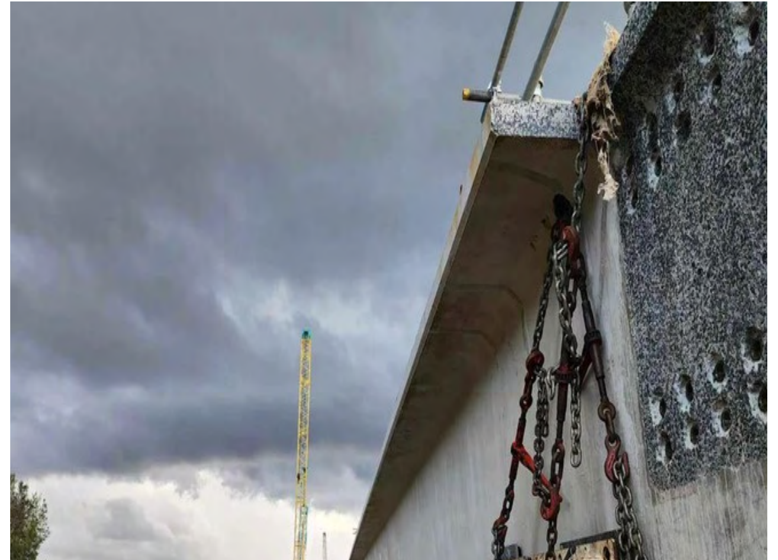
Bridge beam transport capability
