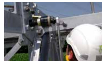
Alkitronic M operating on electricity pylons. Accurate tightening via torque wrench.
