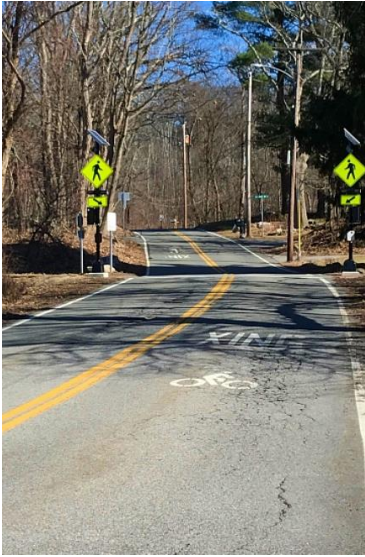
View from High Street showing the newly installed Rapid Rectangular Flashing Beacons
