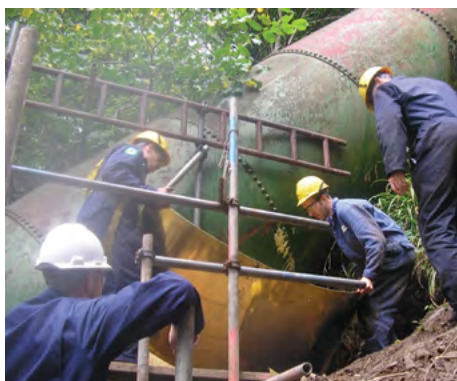
Repair and protection application underway on penstock
