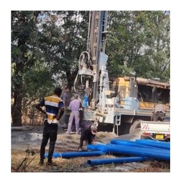
We drilled a 100 meter deep well with a very good yield of water. After successfully completion of drilling and PVC installation we installed a submersible pump, connected the water pipe to the existing raiser and water tank available at Mitimitatu community. Currently, water is now available at the community and can be used for domestic purposes, gardening and supporting other economic activities to generate income and livelihood.
