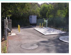
The Village Park 5 Pump Station contains two 15 horsepower pumps, duty and standby, each of which has a pumping capacity of 215 gallons per minute and a 6-inch PVC force main. Bypass piping and valving is available at this pump station to bypass the pump station and utilize the pump station force main. The Village Park 5 Pump Station is also configured with an onsite emergency generator (integral diesel fuel) that autostarts on a loss of SDG&E electrical power or below normal.
