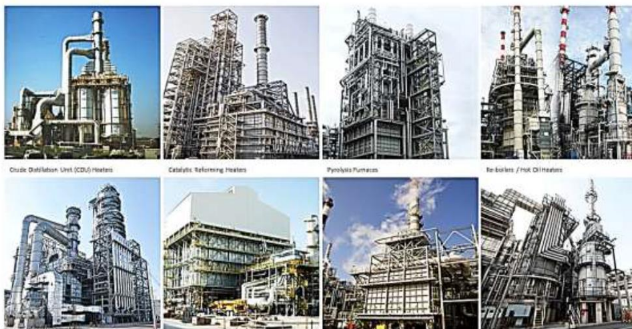
Exhibit 32: Key processes like CDU, VDU, FCCU where fired heaters are used in refineries
