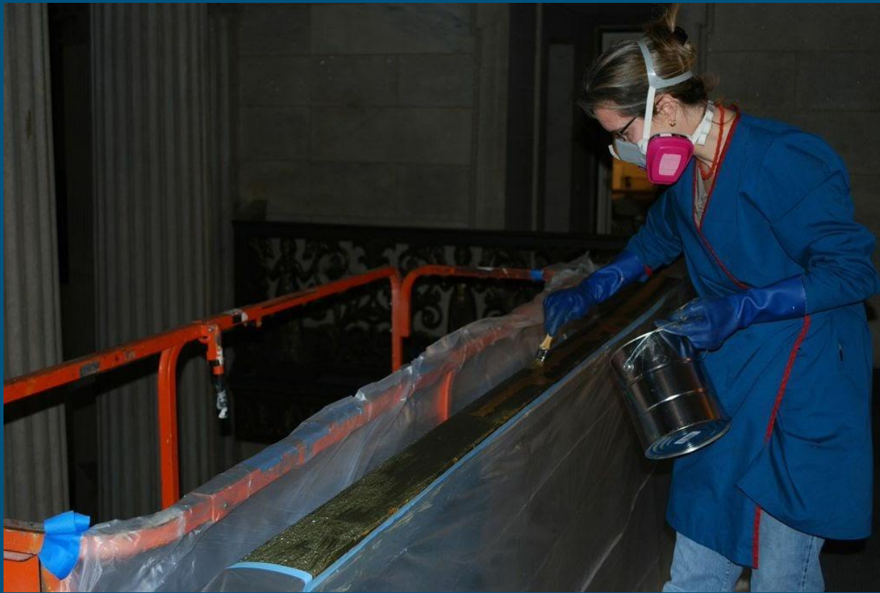
Stripping one of the railings on the upper level balcony
