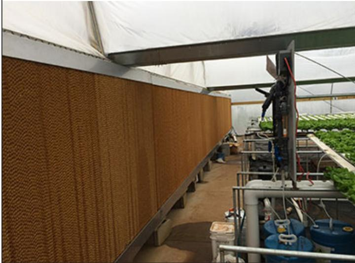
material that is saturated by water dripping over its surface (Figure 27). Excess water is collected in a reservoir and pumped back over the cardboard. Evaporative cooling walls are not efficient in climates with high temperature and high humidity.
