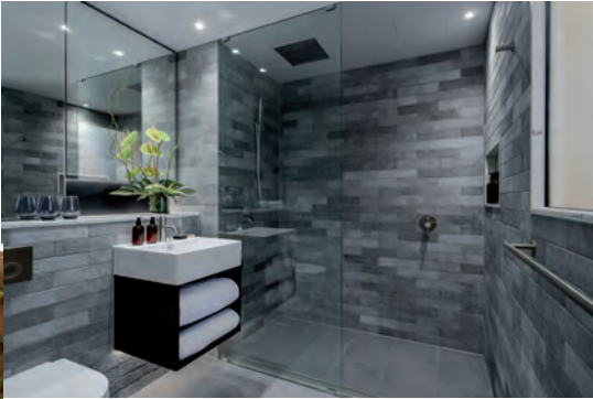
In the bathrooms the screeds were made of TOPCEM, before waterproofing the substrates with MAPEGUM WPS.
