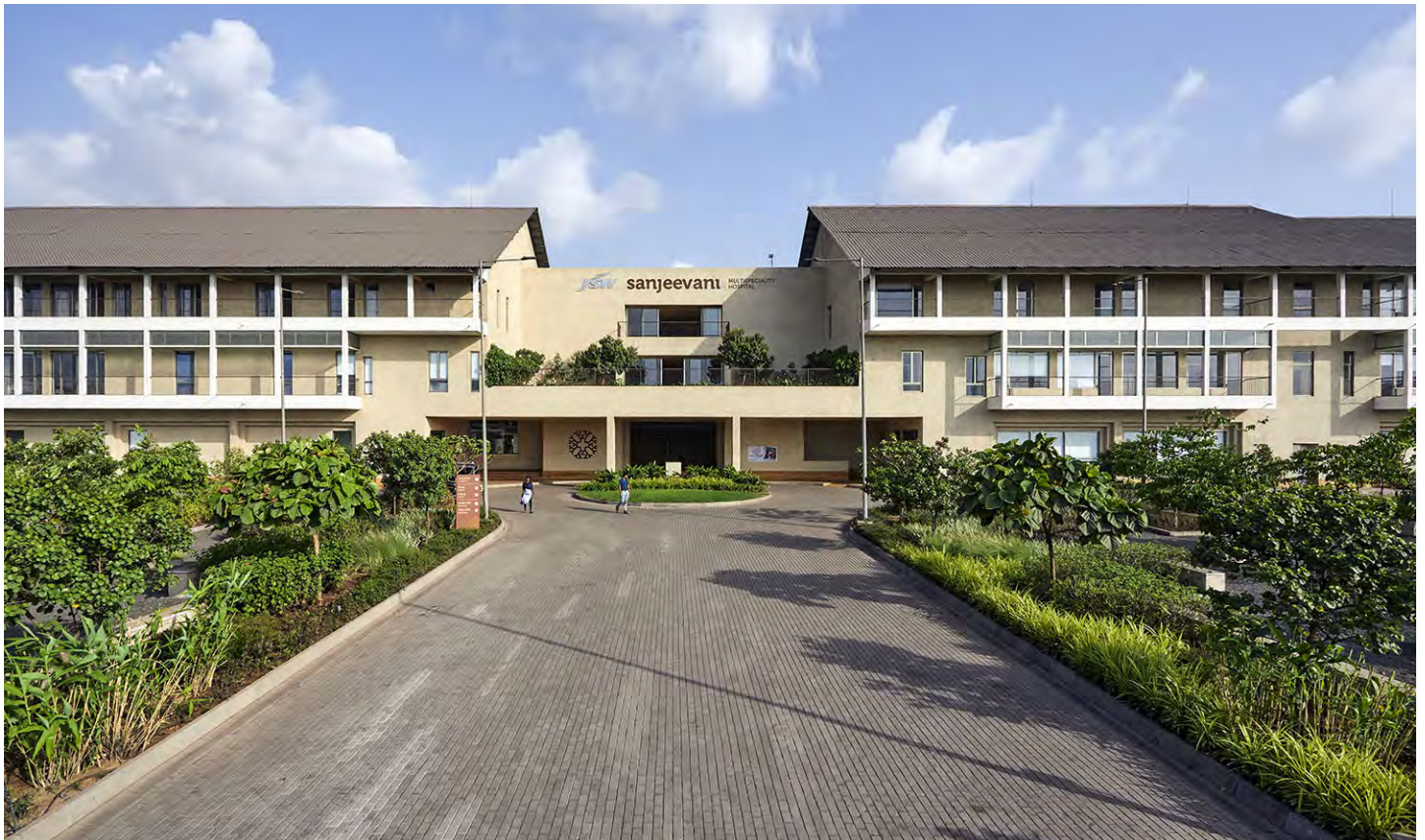
JSW Sanjeevani Multispeciality Hospital in Dolvi, Maharashtra, India, designed by SJK Architects. (Photo copyright: Rajesh Vora)
