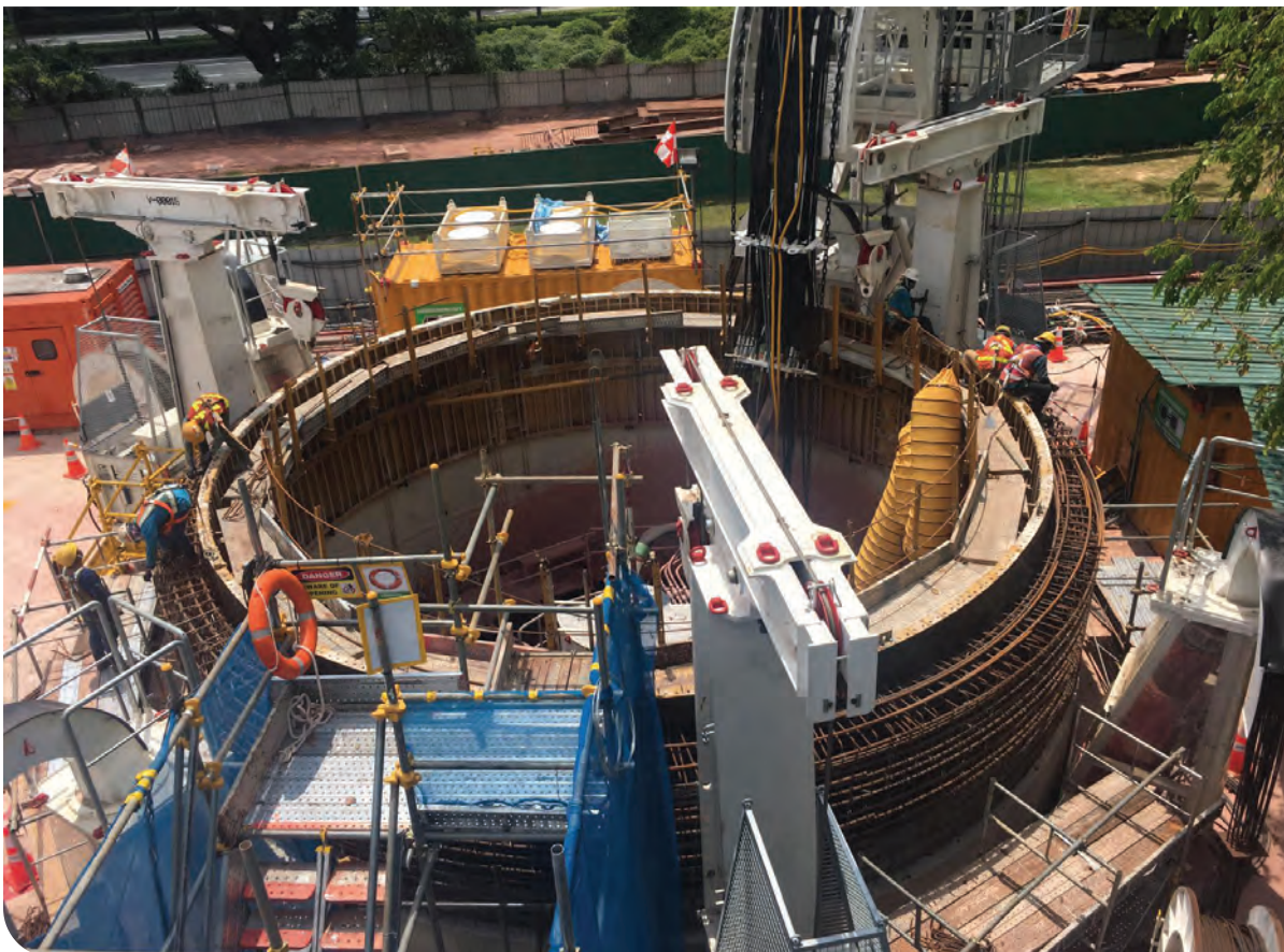
ABOVE AND LEFT: The vertical shaft sinking machine (VSM) technology was used in the DTSS2 T-11 section, allowing safe and quick shaft construction in difficult ground conditions below groundwater table.
