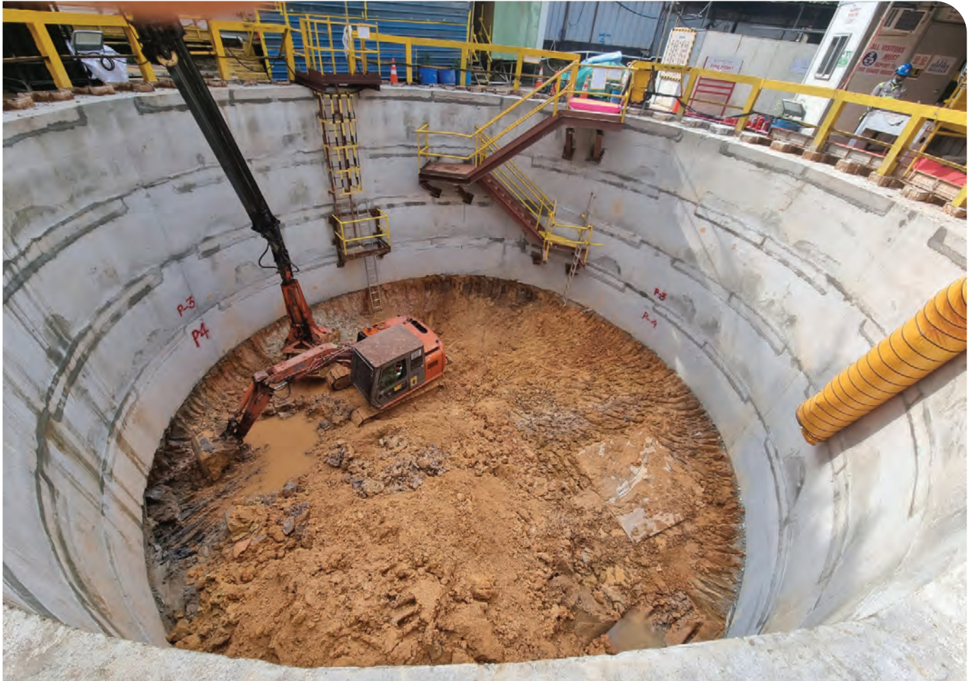
ABOVE AND LEFT: The vertical shaft sinking machine (VSM) technology was used in the DTSS2 T-11 section, allowing safe and quick shaft construction in difficult ground conditions below groundwater table.
