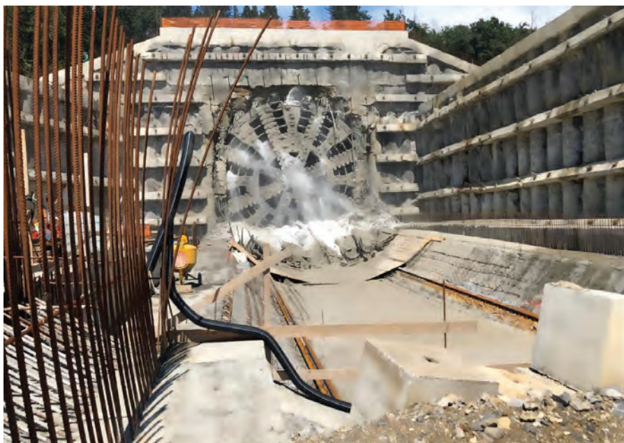
The Polyfoamer Eco 100 Plus foaming agent was used in the EPB TBM to bore the Santa Lucia Tunnel in central Italy, the longest three-lane tunnel in Europe.
