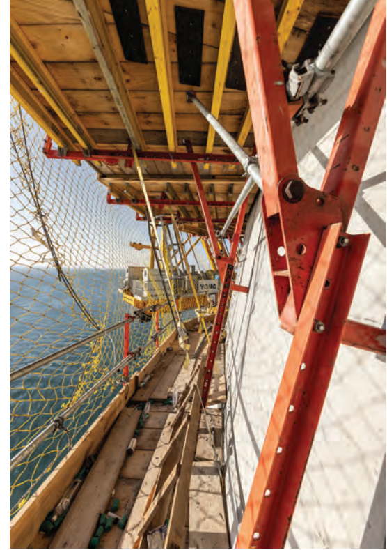
Peri's SCS Climbing System facilitates safe working processes in the lower and upper sections of the pylon.
