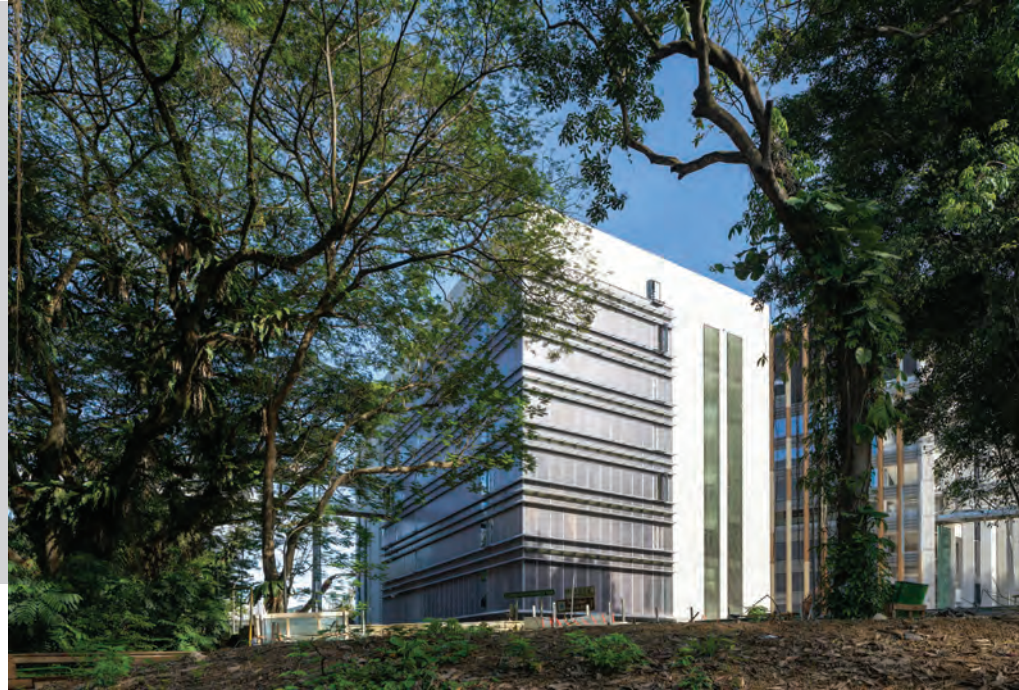
JTC's eight-storey mass engineered timber (MET) building is the tallest timber industrial building in Singapore.
