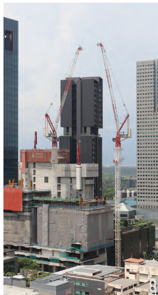
ALL IMAGES: The J480PA tower cranes on the Shaw Tower project. Designed with a compact footprint of 2.16 m, these cranes are ideal for jobsites with limited space. Their boom can be configured in 5-m increments, allowing for customisation based on project requirements.
