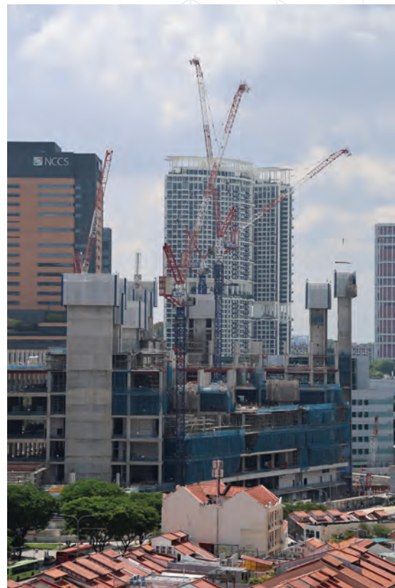
ABOVE AND LEFT: Jaso's J480PA and J380PA tower cranes are deployed at a jobsite in Outram Park, helping to build new medical facilities.
