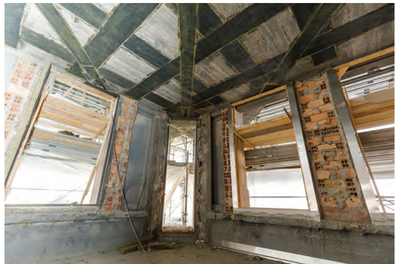
TOP, ABOVE AND ABOVE RIGHT: Structural strengthening work at Torre Velasca skyscraper in Milan, Italy aimed to improve the mechanical properties of the chains and tie rods in the upper floors. The Mapei FRP system was employed here, helping to ensure minimum intrusion on the architecture of the building, increased structural capacity and high durability.
