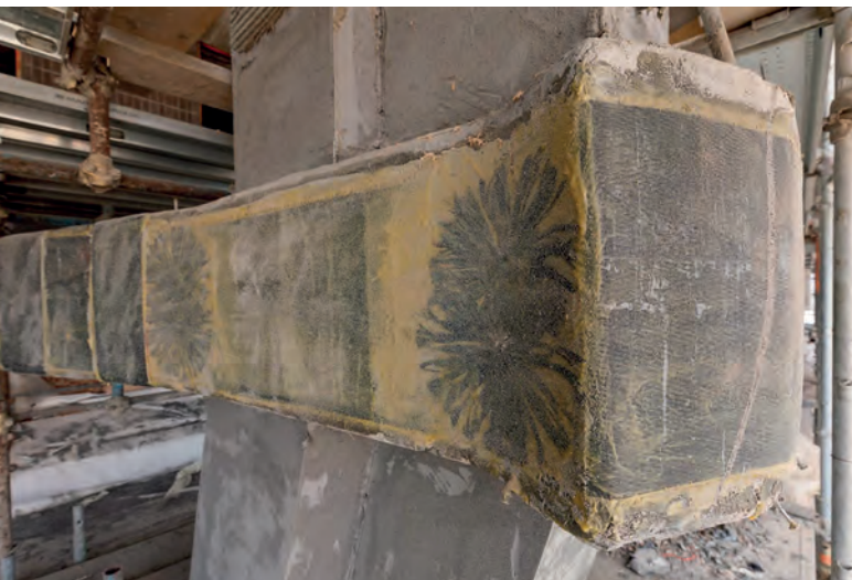
TOP, ABOVE AND ABOVE RIGHT: Structural strengthening work at Torre Velasca skyscraper in Milan, Italy aimed to improve the mechanical properties of the chains and tie rods in the upper floors. The Mapei FRP system was employed here, helping to ensure minimum intrusion on the architecture of the building, increased structural capacity and high durability.
