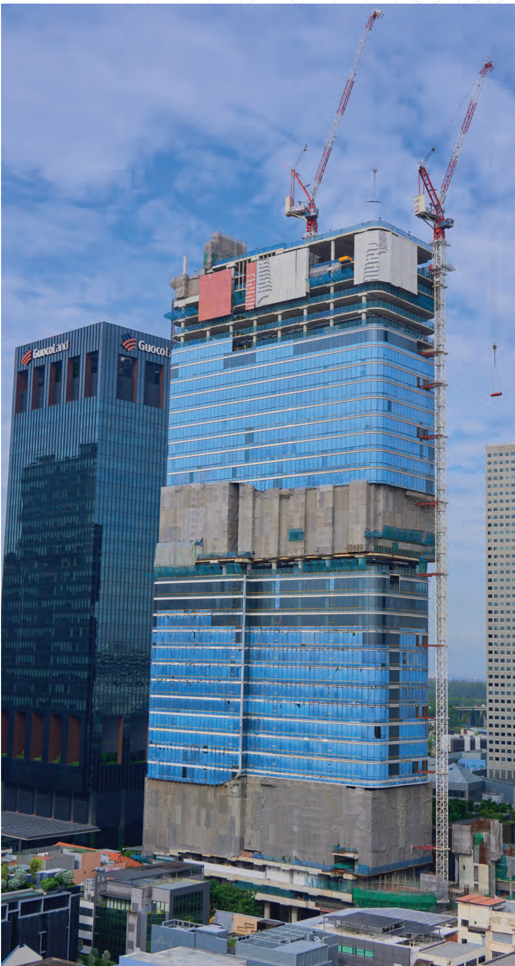
ALL IMAGES: The J480PA tower cranes on the Shaw Tower project. Designed with a compact footprint of 2.16 m, these cranes are ideal for jobsites with limited space. Their boom can be configured in 5-m increments, allowing for customisation based on project requirements.
