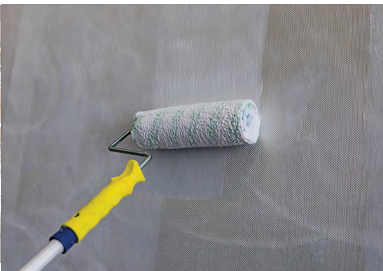
TOP, ABOVE AND ABOVE RIGHT: For this building, the MapeWrap EQ system was applied to prevent walls from brittle breaking and overturning in the case of a seismic event.
