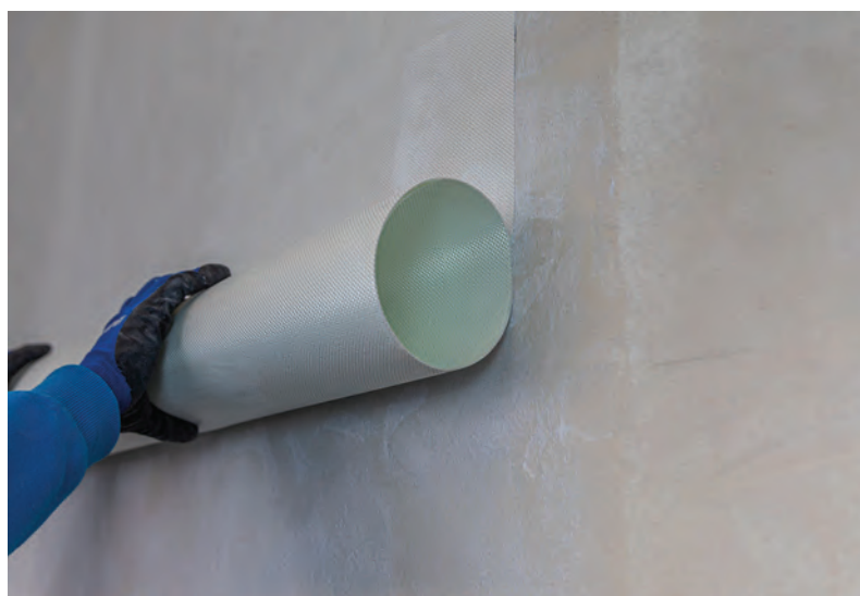
TOP, ABOVE AND ABOVE RIGHT: For this building, the MapeWrap EQ system was applied to prevent walls from brittle breaking and overturning in the case of a seismic event.
