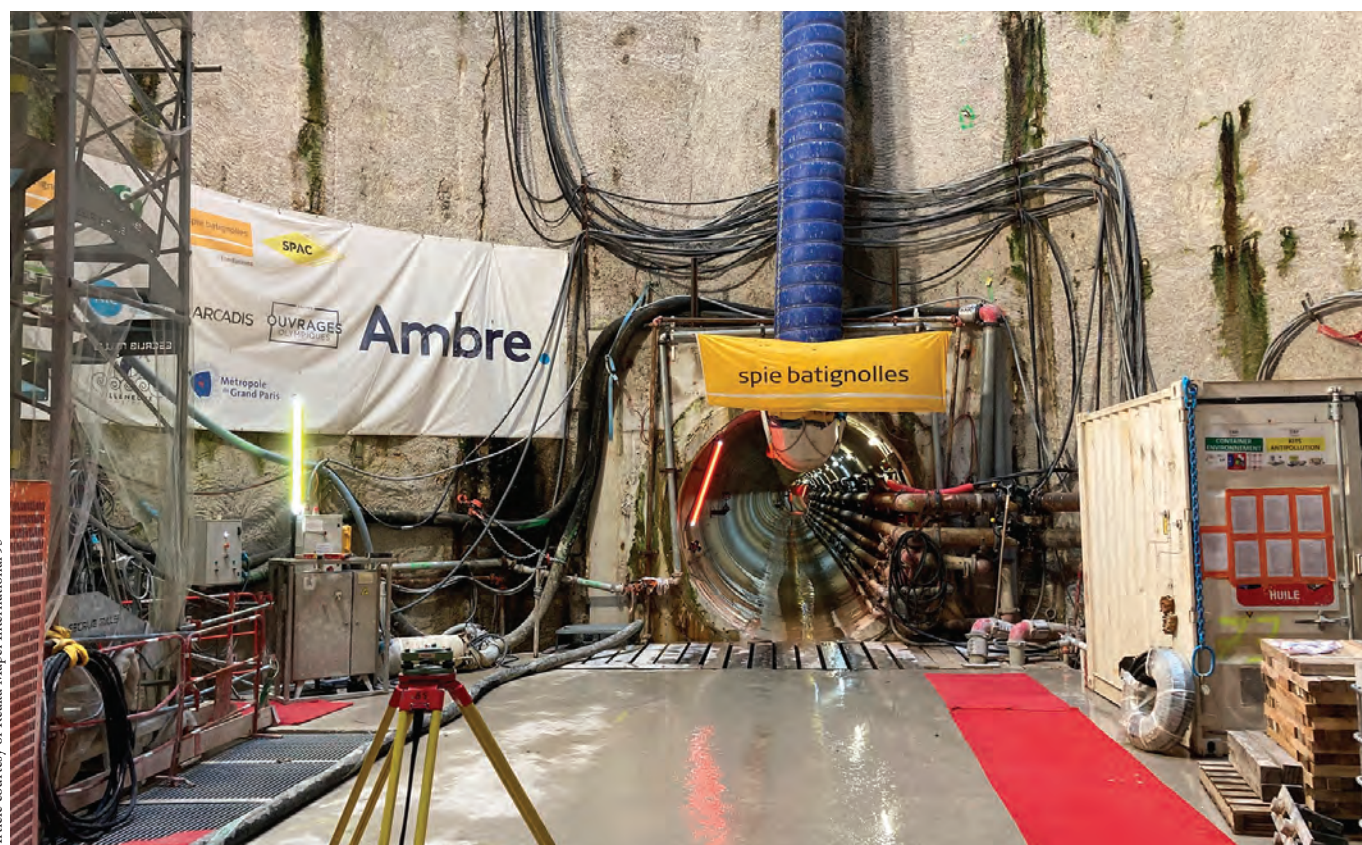
TOP: Mapei was engaged to supply its products for injections and TBM works. The company's two-component system is considered the most suitable for this site. ABOVE: At a depth of 50 m, the tunnel is approximately 2.5 km long and 3 m in diameter. The entrance to the tunnel can be seen here.
