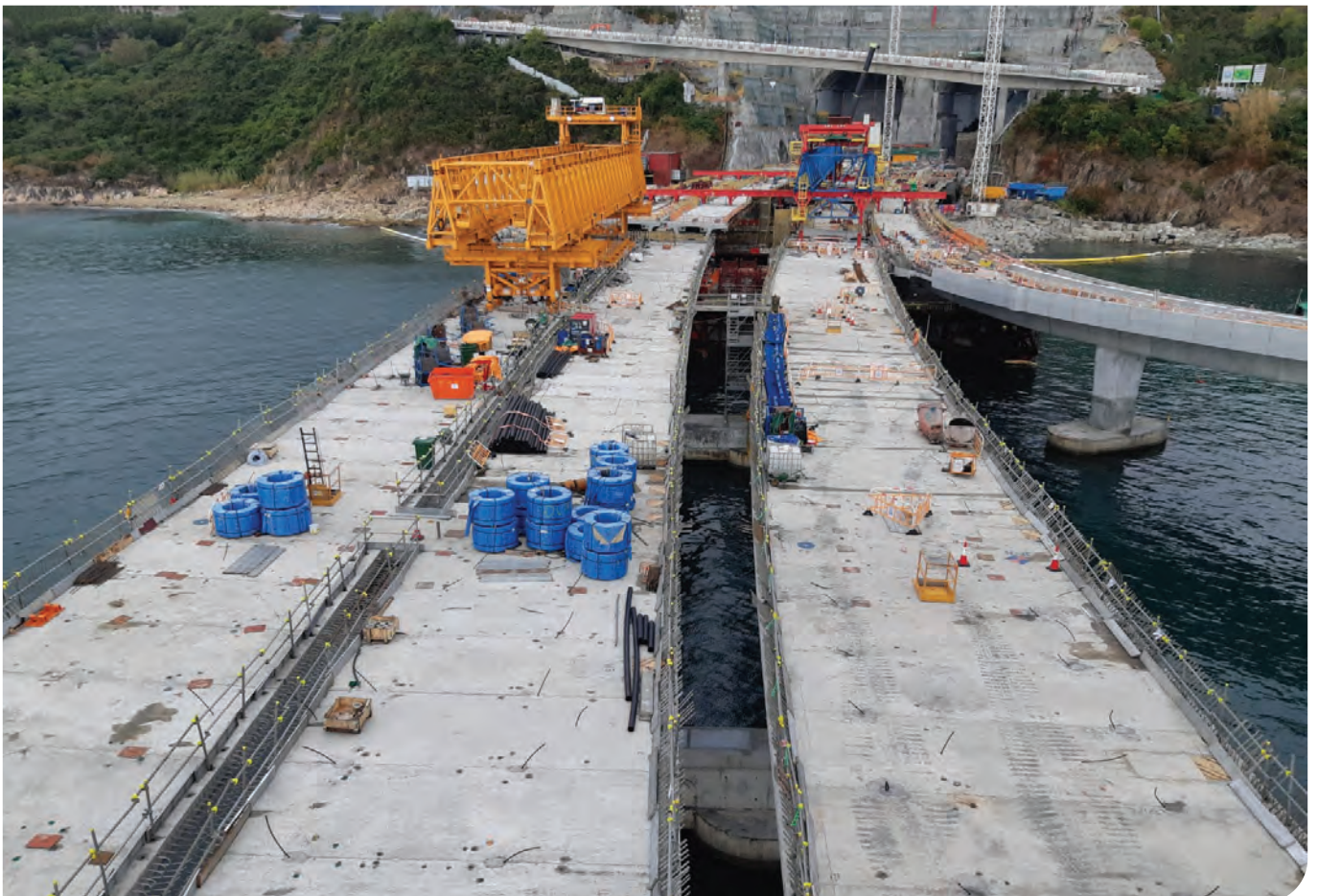
This new elevated interchange over the sea, which consists of seven post-tensioned concrete bridges, was erected using the precast segmental balanced cantilever method.
