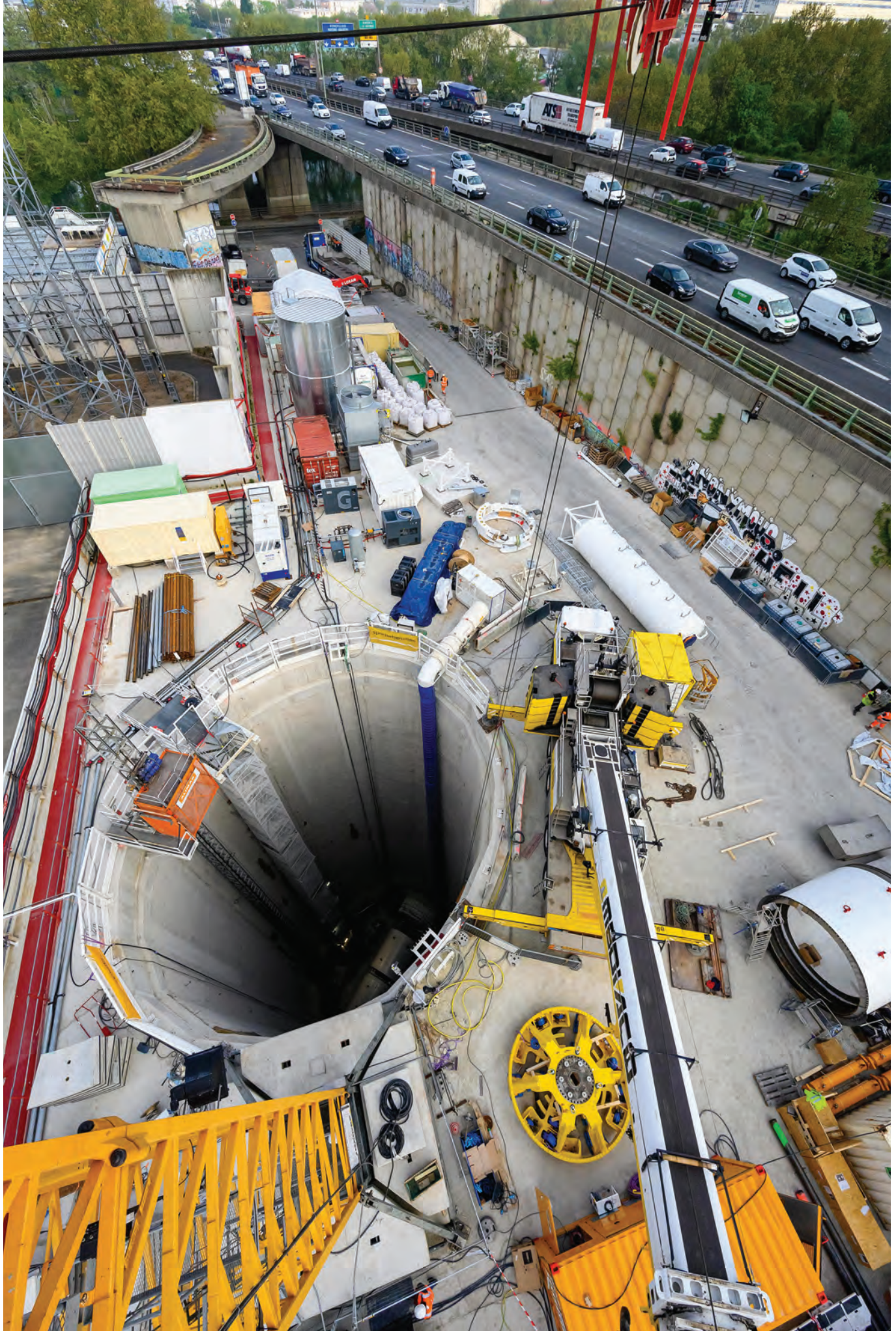
OPPOSITE AND ABOVE: Excavating the tunnel with a 120-m-long TBM called Ambra. The work required a total of 120,000 liner segments to be installed. When completed, the new tunnel will be used to run powerlines underground.
