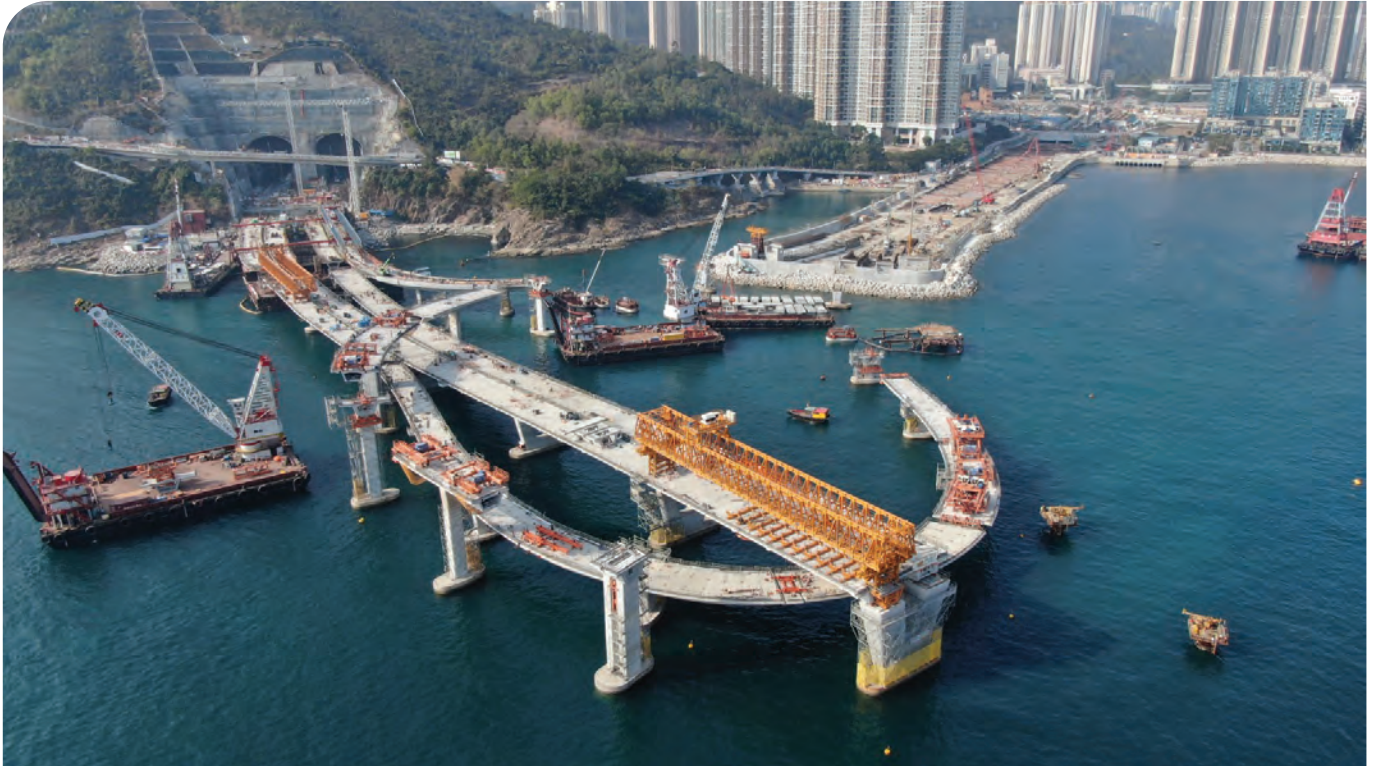
Aurecon was commissioned to deliver structural, geotechnical and temporary design works for the bridge component of the TKO Interchange and Associated Works project.
