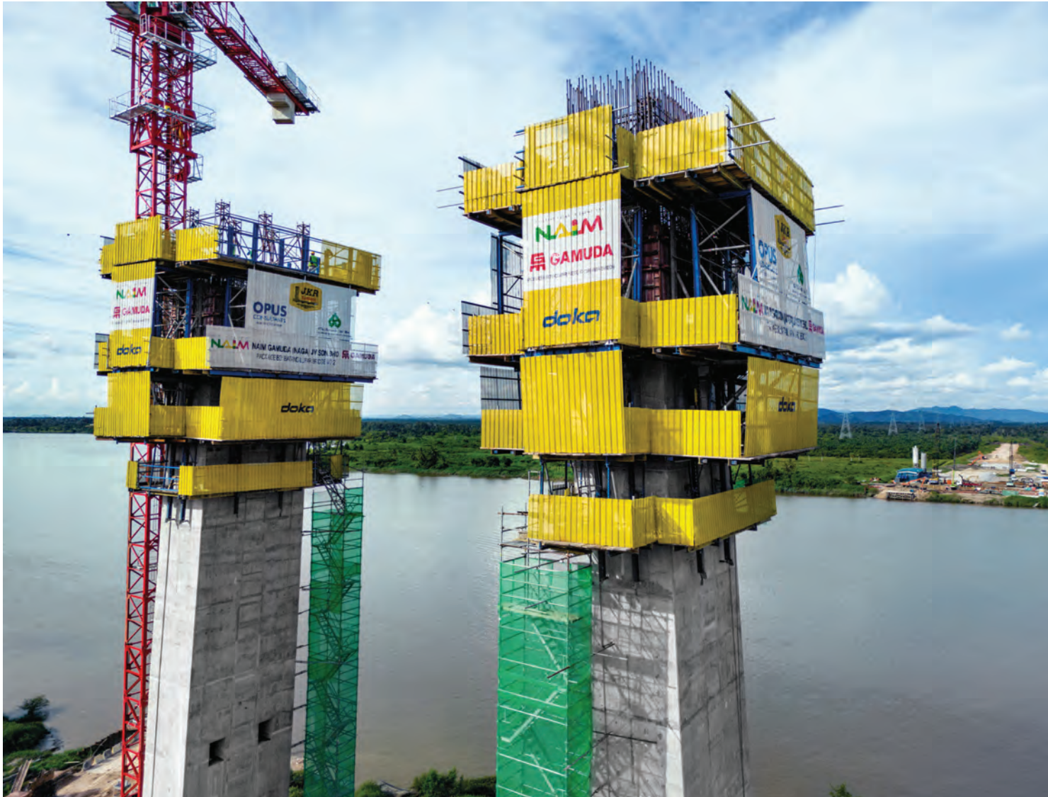
Doka's Automatic Climbing Formwork SKE 100 plus has already saved months from the project schedule.
