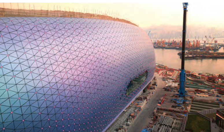
LEFT AND RIGHT: The main stadium facade consists of approximately 27,000 triangular aluminium panels.
