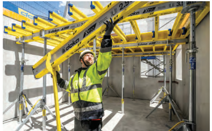
Doka XT20 beam (above) and Doka Eurex 20 basic floor prop (below).
