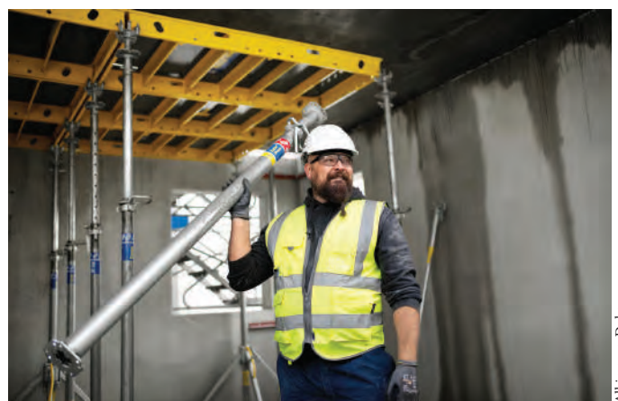
Doka XT20 beam (above) and Doka Eurex 20 basic floor prop (below).
