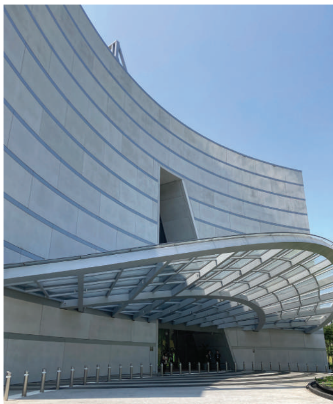
LEFT AND BELOW: The main entrance is a key engineering complexity in SJ Campus. It features a large glass canopy, up to 16 m in length (with a span-depth ratio of 1:40), without any support of conventional tiebacks, thus requiring sophisticated parametric analysis.
