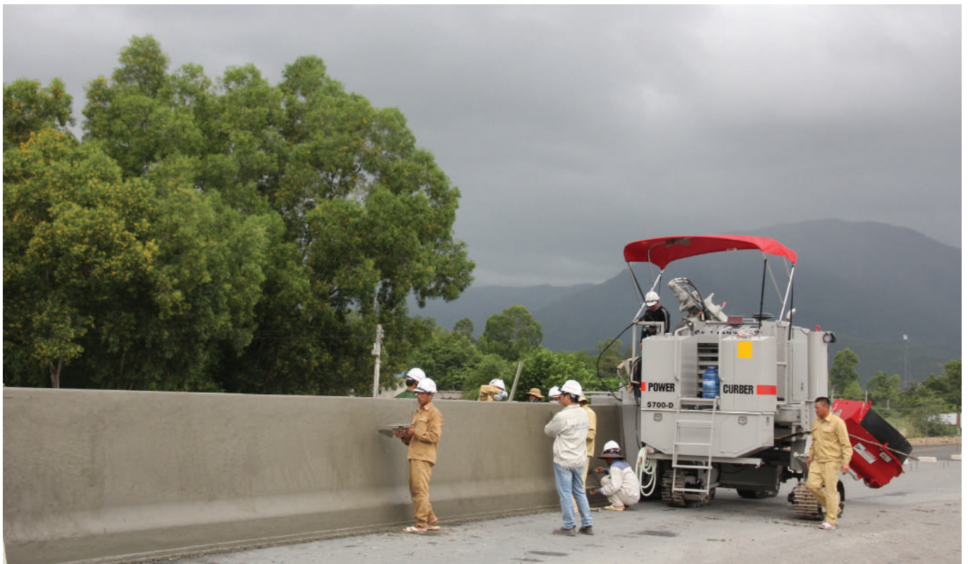
ABOVE AND BELOW: This is said to be the first time a slipform machine has poured a barrier wall in Vietnam. The Power Curber 5700-D has been working on several sections of the expressway, operating three shifts per day.
