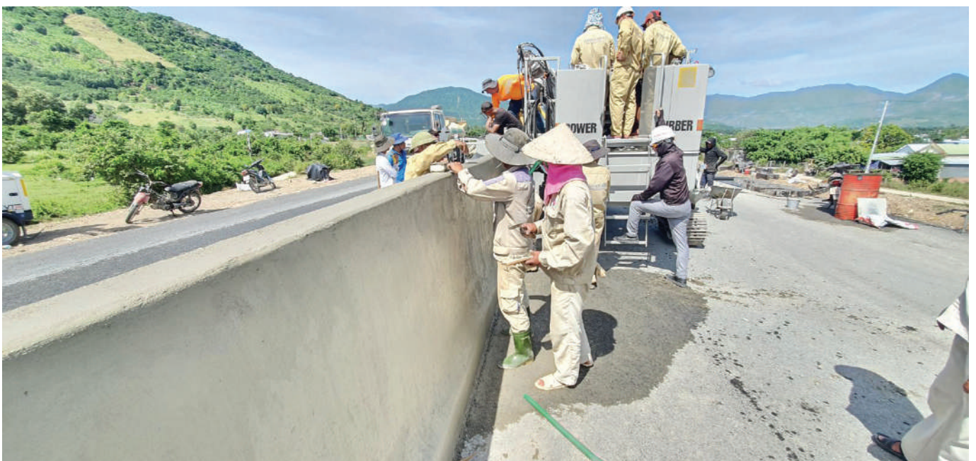
TOP AND ABOVE: The North-South Expressway is Vietnam's most important transportation corridor, with some sections still under construction. A Power Curber 5700-D slipform machine is being used by road contractor Son Hai to slipform safety barrier walls, increasing the quality and speed of production for this major infrastructure project.
