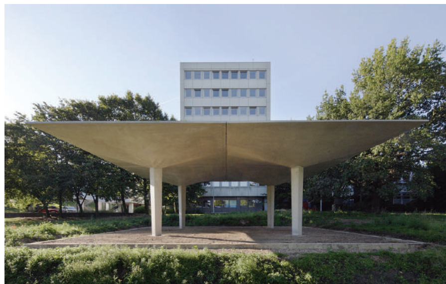
Picture from the construction of a pavilion at the RWTH Aachen University of Technology, Germany. The shell-shaped roof structure has been reinforced with carbon fibre textile and is only 6 cm thick.
