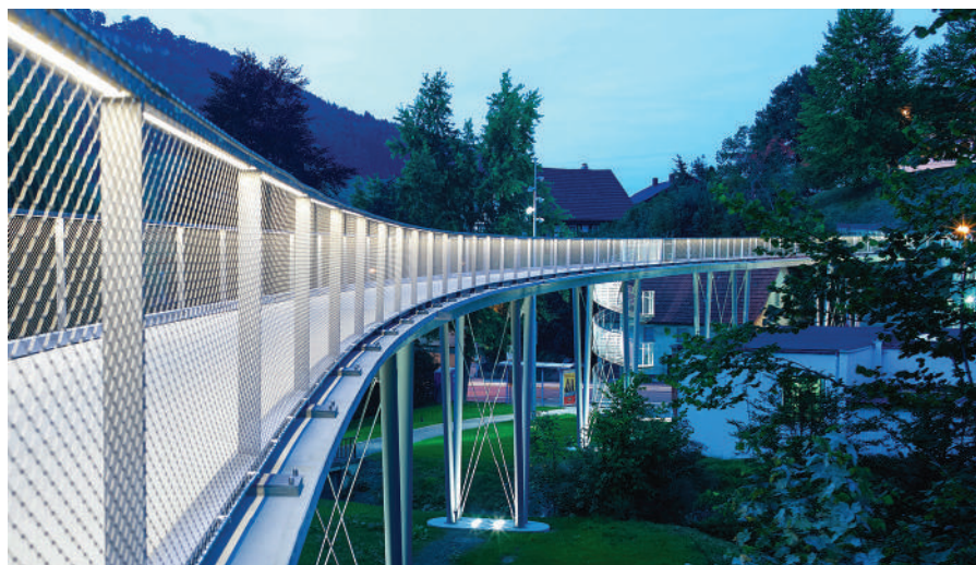
The pedestrian and bicycle bridge in Albstadt, Germany, is an early example of a textile-reinforced concrete structure. The bridge is about 100 m long.
