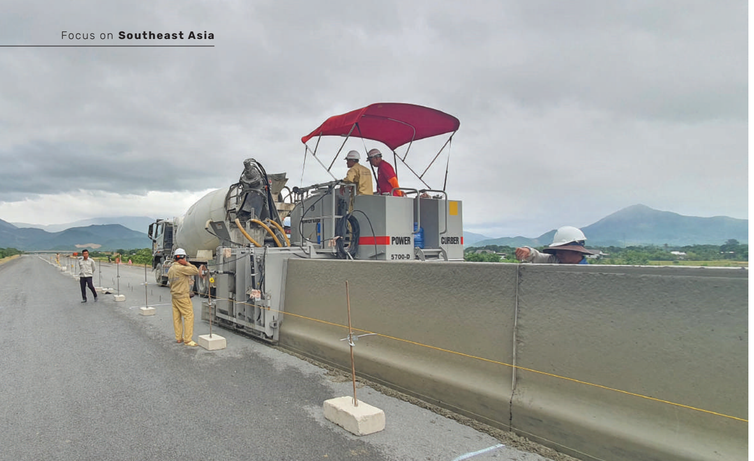
ABOVE AND BELOW: This is said to be the first time a slipform machine has poured a barrier wall in Vietnam. The Power Curber 5700-D has been working on several sections of the expressway, operating three shifts per day.
