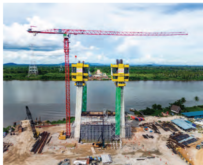
Doka was also engaged to provide a flexible formwork solution for the cable-stayed Batang Lupar Bridge No. 2 in Sarawak, Malaysia, in particular to cater to the unusual shape of the pylons.
