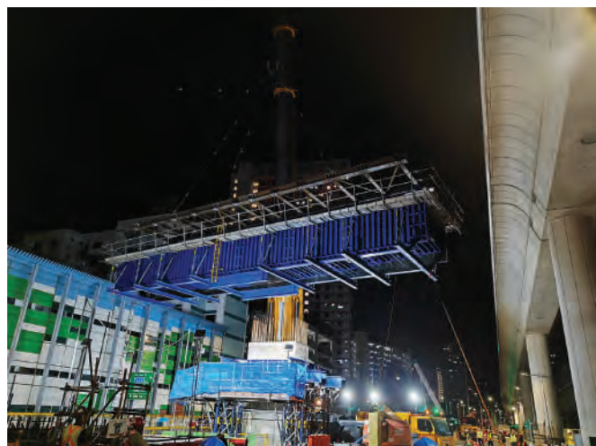
Another major project in which Doka took part was the construction of Jurong Region Line (JRL), Singapore's seventh MRT line. The company supplied its formwork systems for three stations and a viaduct.
