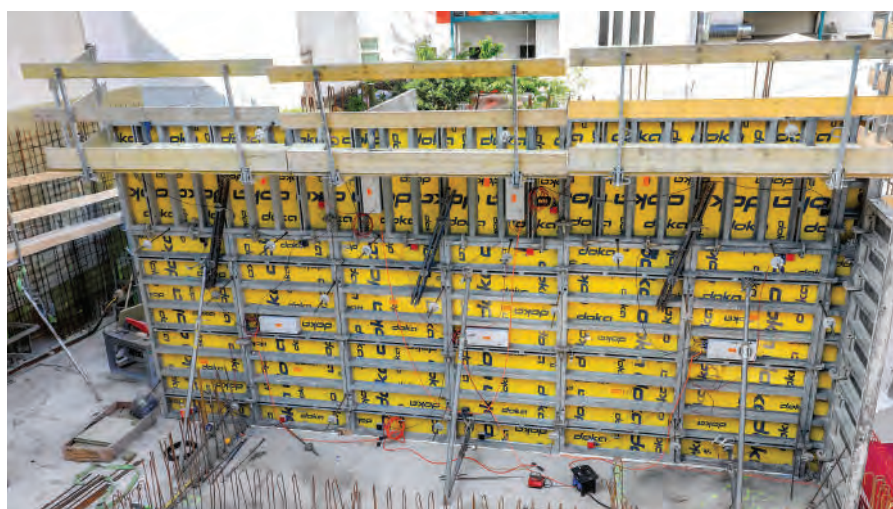
To boost the spread of new, more climate-friendly concrete mixes, Doka has developed an intelligent heated formwork prototype. Through targeted heating, the prototype accelerates the delayed strength development of CO 2 -reduced concrete, enabling safe and efficient use on site.
