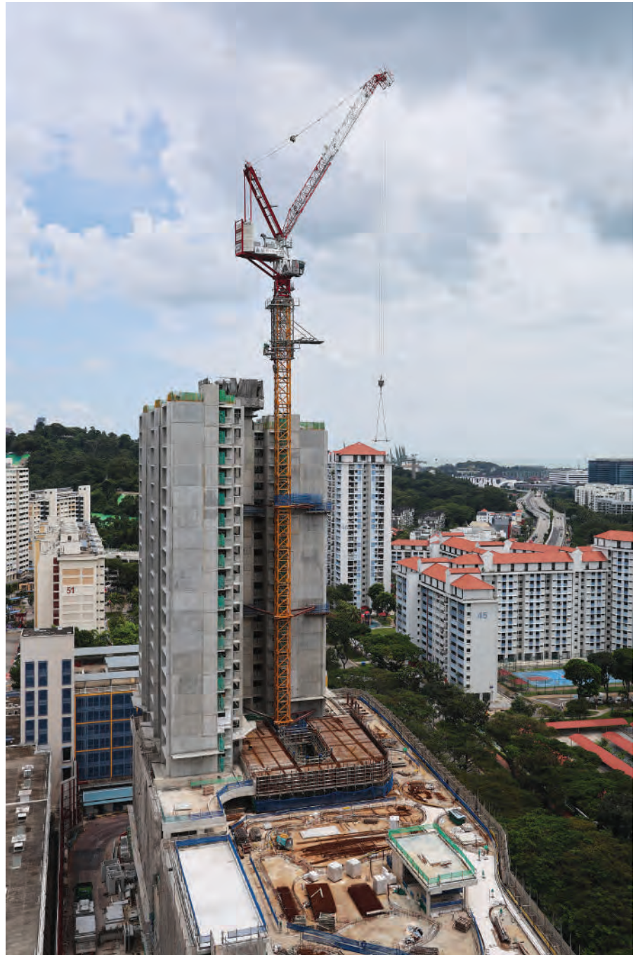
Jaso's J480PA luffing tower crane is designed for high efficiency, safety and versatility on the jobsite, featuring a compact footprint of 2.16 m. This model is available globally, including in Singapore.
