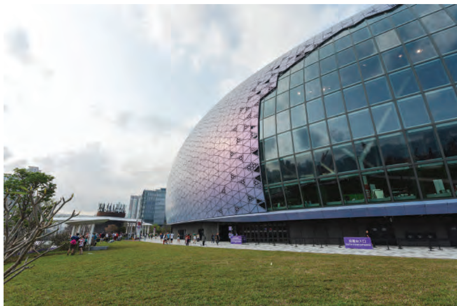
ABOVE: The stadium's facade is composed of around 27,000 triangular aluminium panels that can change into various pearlescent hues depending on the daylight intensity.
