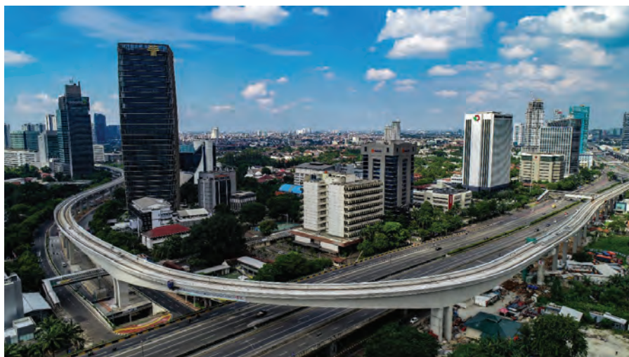
ABOVE AND BELOW: One of the notable features of the project is the U-shape girder system used to construct the viaducts. The slim shape has proved to be an elegant and cost-effective solution, saving space in the dense urban surroundings.
