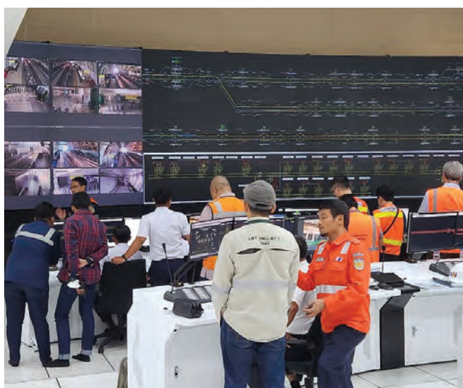
ABOVE AND LEFT: A key consideration for the SMEC team was to oversee the implementation of a reliable automation and communication system. This system, known as Grade of Automation Level 3, transmits information between the train control system, the signalling system and the safety systems.
