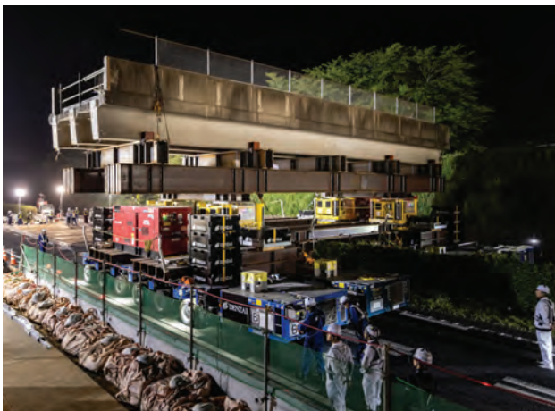
Transporting the bridge to the off-highway rigging location.
