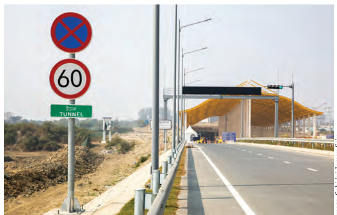
ABOVE: The entrances of the tunnel are built to withstand cyclonic tidal surges that are common in the Bay of Bengal.
