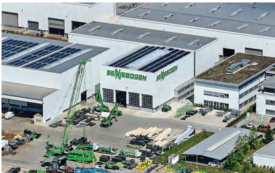
Sennebogen's new product development campus at the Straubing/Port site brings new machine development, testing and prototype construction together in a central location to create synergies and enable a more intensive focus on the development of new technologies.
