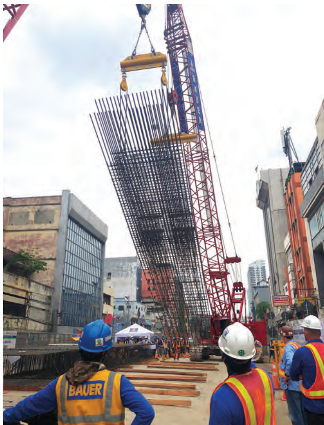
The reinforcement cages were constructed at Bauer Indonesia's workshop and delivered just-in-time to the site.
