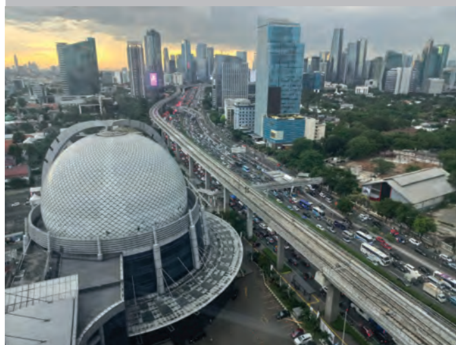
ABOVE AND BELOW: One of the notable features of the project is the U-shape girder system used to construct the viaducts. The slim shape has proved to be an elegant and cost-effective solution, saving space in the dense urban surroundings.
