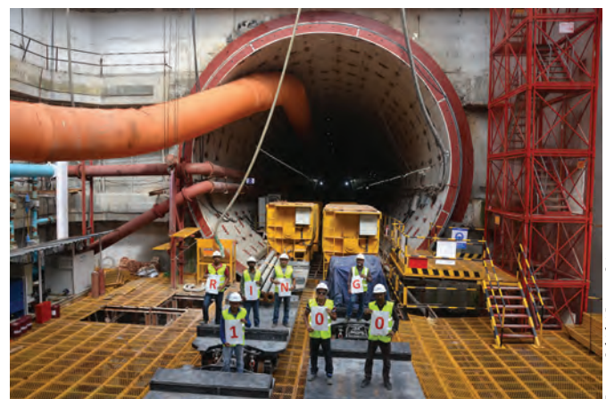
ABOVE: Approximately 1,225 precast concrete rings have been installed to line the tunnel.
