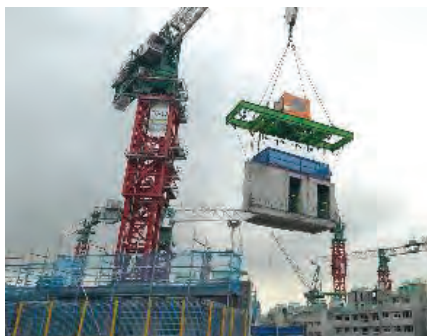
The AI-powered autonomous tower crane with Skyjuster is seen here lifting and transporting a precast module.
