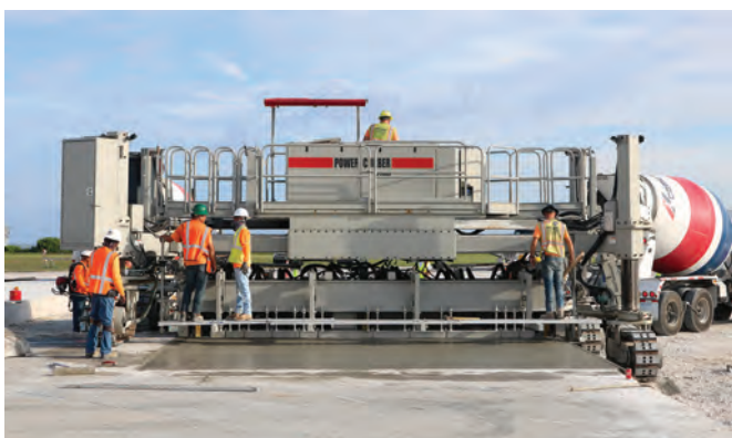
The Power Curber 7700 multipurpose slipform machine is designed for a wide variety of offset and paving applications.
