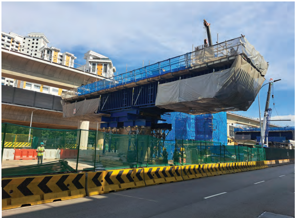
ABOVE: Following just one night of road closures, Doka's Steel Girder Formwork and UniKit shoring tower ensured a key stage of the Toh Guan Station was completed on time and on budget.
