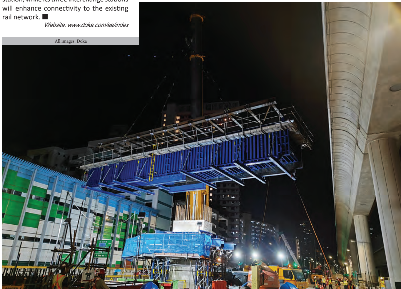
BELOW: Doka's solution included crane-lifting its Steel Girder Formwork at night to avoid disruption to existing infrastructure.
