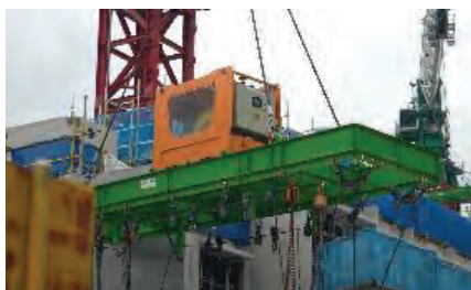
The integration of the Skyjuster to the lifting frame helps eliminate swaying motions of the modules, and automate the rotation and positioning of suspended components to the intended alignment before they are lowered into place.
