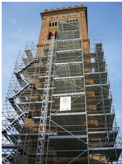
LEFT, MIDDLE AND RIGHT: Tendo designs and manufactures steel scaffolding systems for industrial and construction applications. The company provides two scaffolding models – frame and multi-directional – which are inter-compatible in terms of height.
