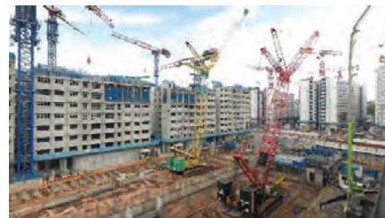
With the crane machine guidance technology, two mobile cranes can be safely deployed side by side within a confined space.
