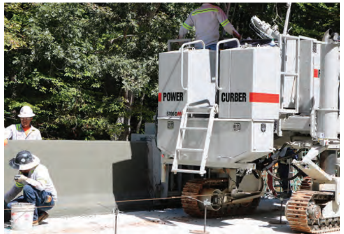
The Power Curber 5700-D curb & gutter machine is a 'one-machine solution' that can easily handle curb & gutter work, highway safety barriers, irrigation ditches, sidewalks and other special applications.
