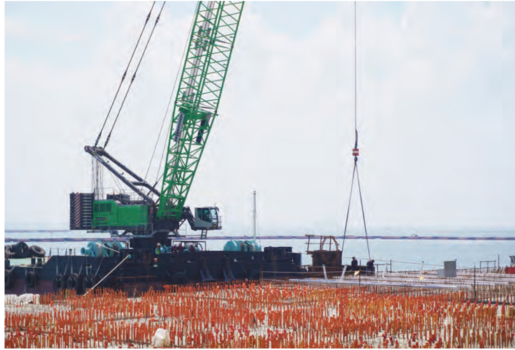
RIGHT: A Sennebogen 6300E duty cycle crane with a lifting capacity of up to 300 t being used in the expansion project.
