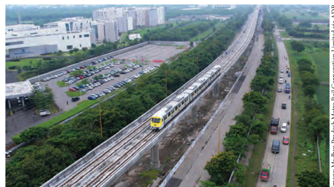
The Indore Metro Rail Project is expected to significantly reduce greenhouse gas emissions – by an estimated 12,414 t of carbon dioxide equivalent annually – and improve air quality in one of India's fastest-growing urban centres.
