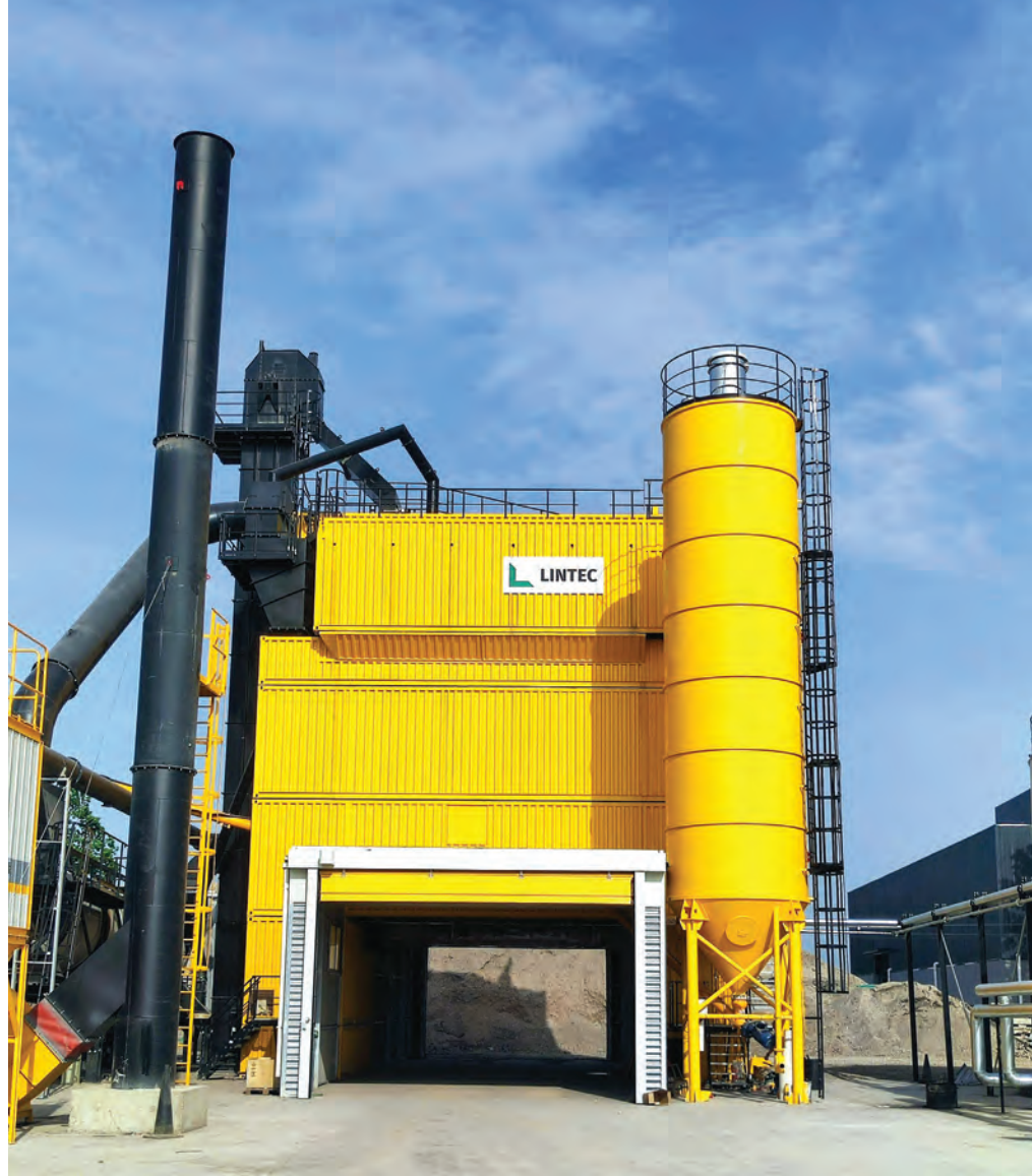
ABOVE AND BELOW: With a 240 t/hr capacity, the CSM3000 plant has already produced nearly 10,000 t of premium asphalt mix. Delivered as a complete turnkey project, the Lintec & Linnhoff team oversaw every stage of the process, from plant transportation and installation to commissioning and operator training.
