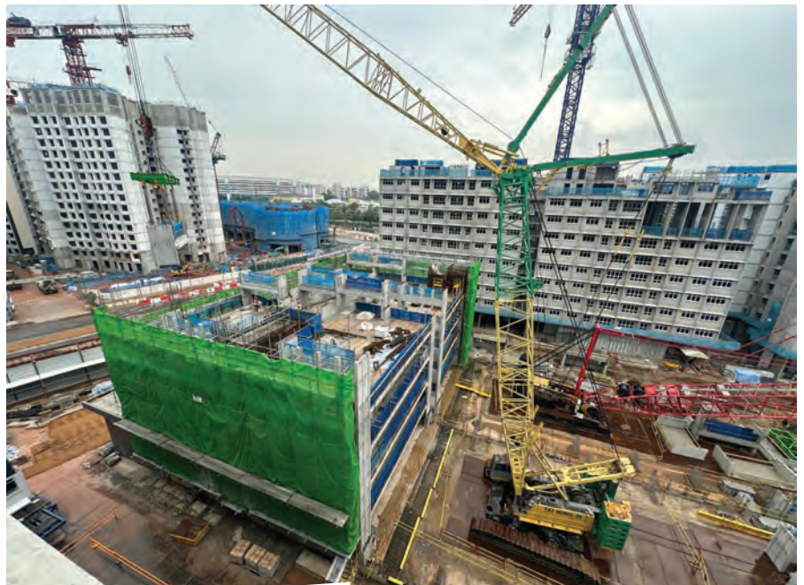
ABOVE AND LEFT: Obayashi has deployed its autonomous tower crane and machine guided crawler crane in Singapore. These solutions aim to increase productivity, improve safety and reduce reliance on manpower.
