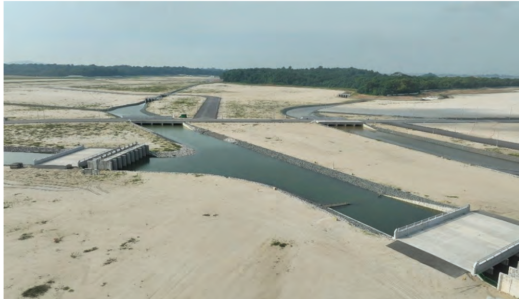
ABOVE: During dry weather, water is recirculated by pumping water from the stormwater collection pond to the polder drainage network (pictured) to prevent stagnation.
