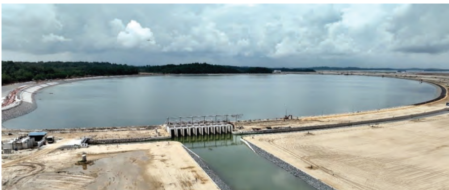
When it rains, runoff within the polder and the Pulau Tekong catchment area is conveyed to the 116-ha stormwater collection pond (pictured) to mitigate flooding within the polder.
