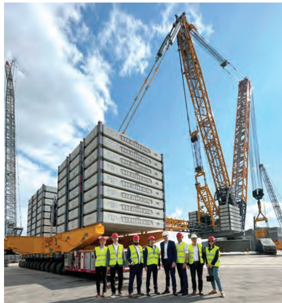
LEFT: Denzai and Liebherr representatives, with the new 2,500-t Liebherr LR12500-1.0 crawler crane.
