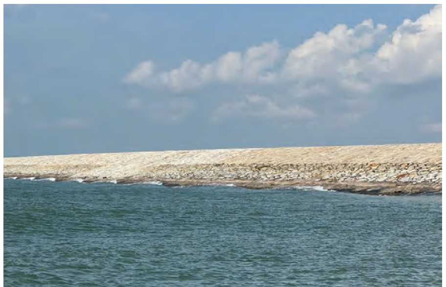
TOP: A 10-km-long coastal dike protects the low-lying polder land from the sea. Natural materials are used on both sides of the coastal dike.
