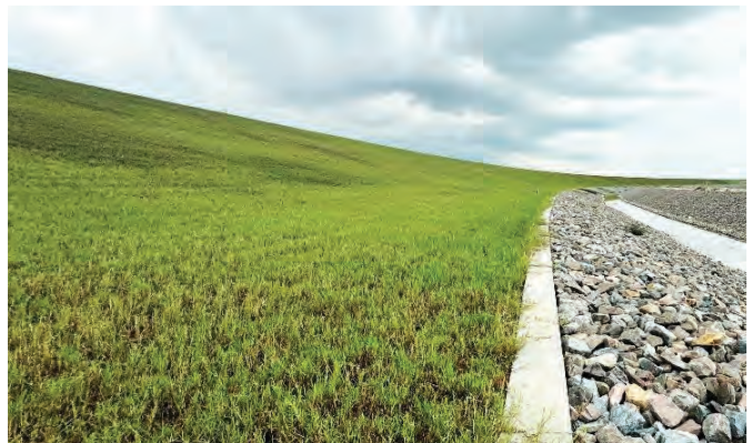
Bermuda grass covers the landward side of the coastal dike to mitigate erosion, while beautifying the landscape.
