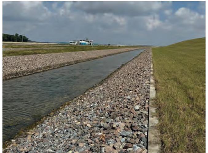
The seepage drain on the landward side of the coastal dike.
