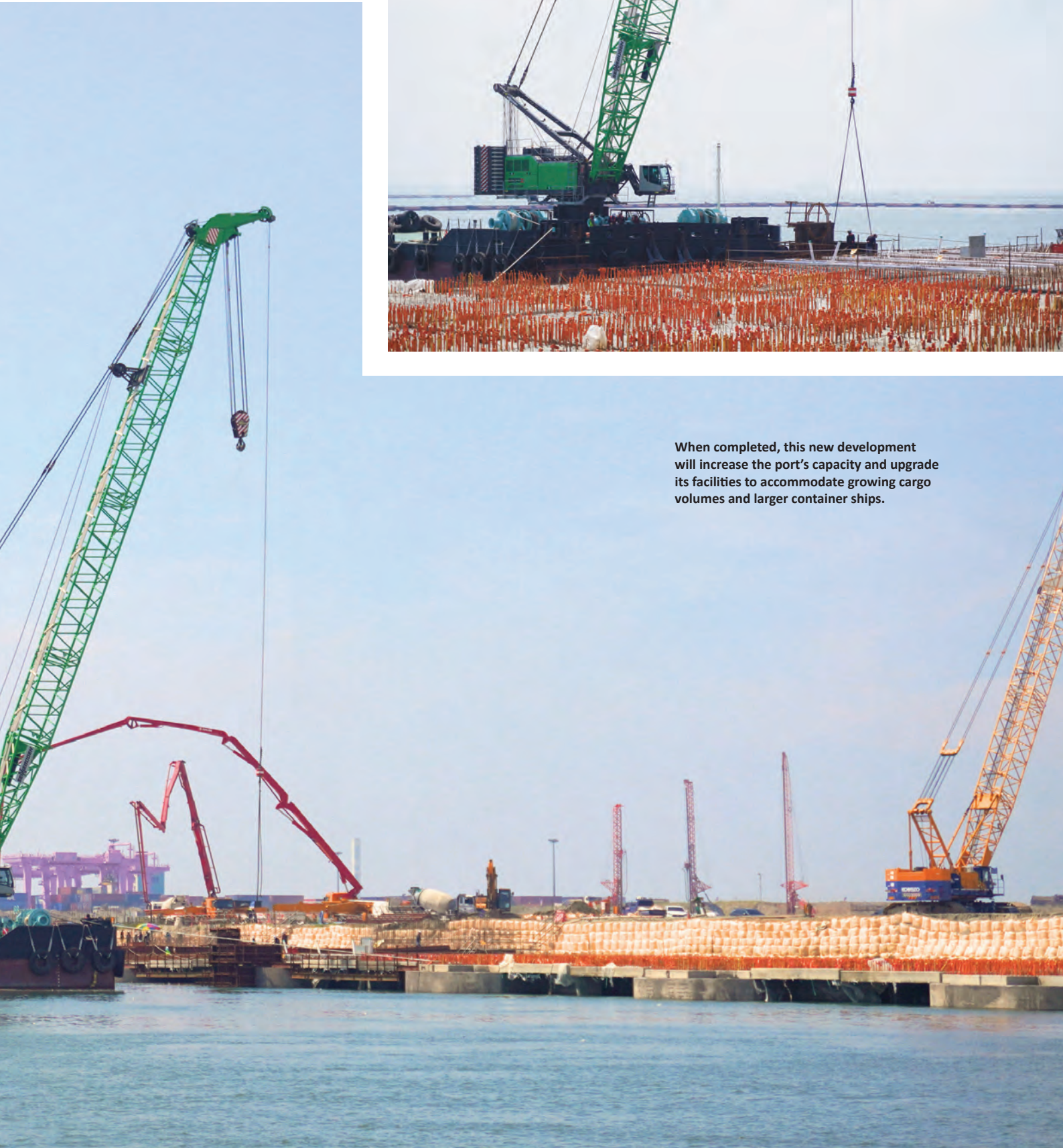
RIGHT: A Sennebogen 6300E duty cycle crane with a lifting capacity of up to 300 t being used in the expansion project.
