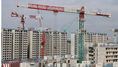
LEFT AND RIGHT: Jaso's J1400 tower cranes have recently been deployed on a residential project in Singapore, which was built using the PPVC (prefabricated prefinished volumetric construction) method. With a maximum 80-m-long jib, the J1400 can lift a maximum load of 64 t.
