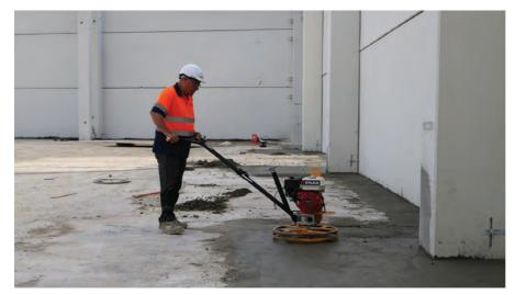
Enar also offers concrete finishing solutions such as trowels (above), and compaction equipment, including tamping rammers (right).
